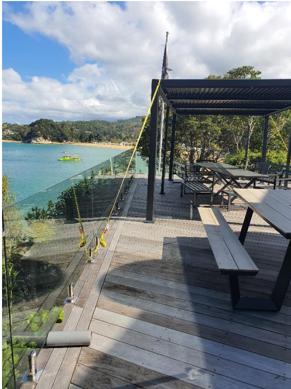
Photo H: Deck towards the west, showing glass balustrade.
