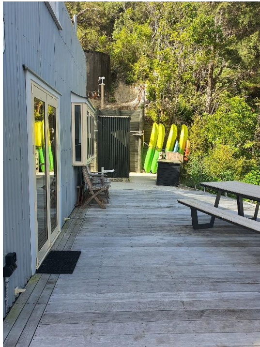
Photo G: Deck that has been erected from the southern corner of the dwelling towards the east.
