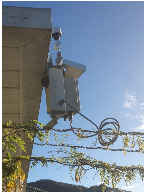
Figure 3: Photograph of one of the ES642 units being installed in Murchison.
