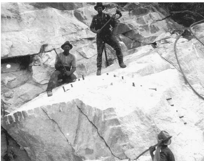
Blocks of marble are cut at Kairuru quarry in the 1920s. Small holes were drilled and wedges inserted. (Alexander Turnbull Library, Lithgow Collection)
