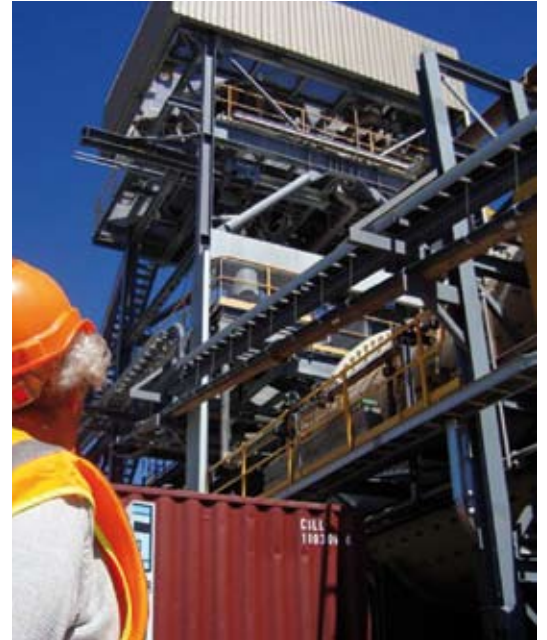
The huge grinding plant processes quartz rock.
