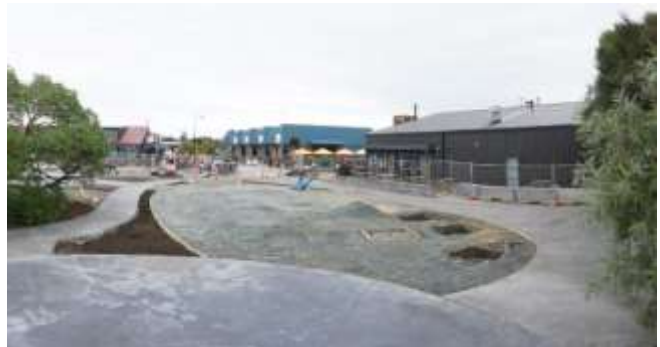
Hard landscaping underway, June 2021
