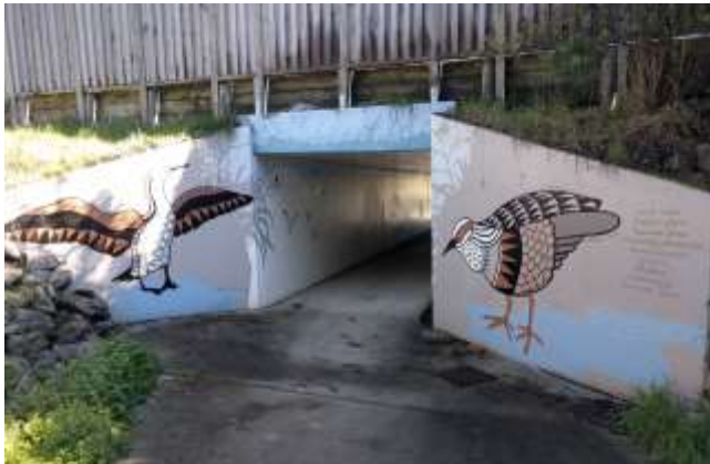
Highway underpass just east of the walkway.
