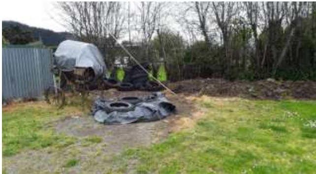
Encroachment into the reserve parcel that adjoins Wakefield Bowling Club
