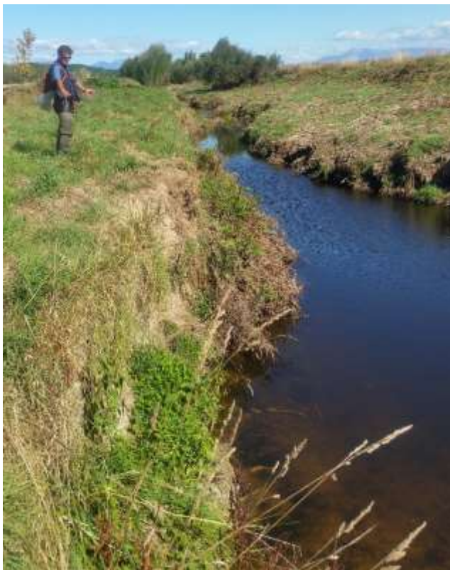
Left: Company Ditch No1 approximately 300m upstream of Wilson Road. Shows the removal of shrubby willow. Replanting in mixed natives and shrubby willow would achieve good shading through this section.
