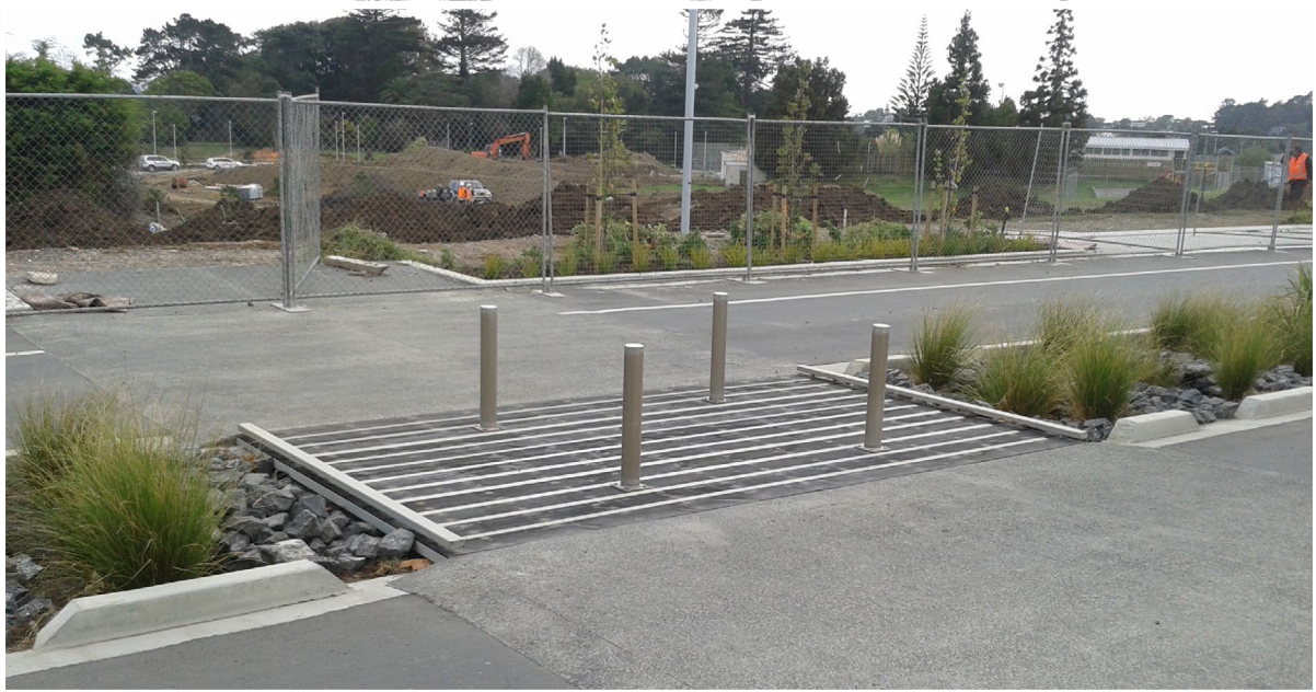
Figure 18. Stormwater infrastructure and street design, Hobsonville, Auckland
