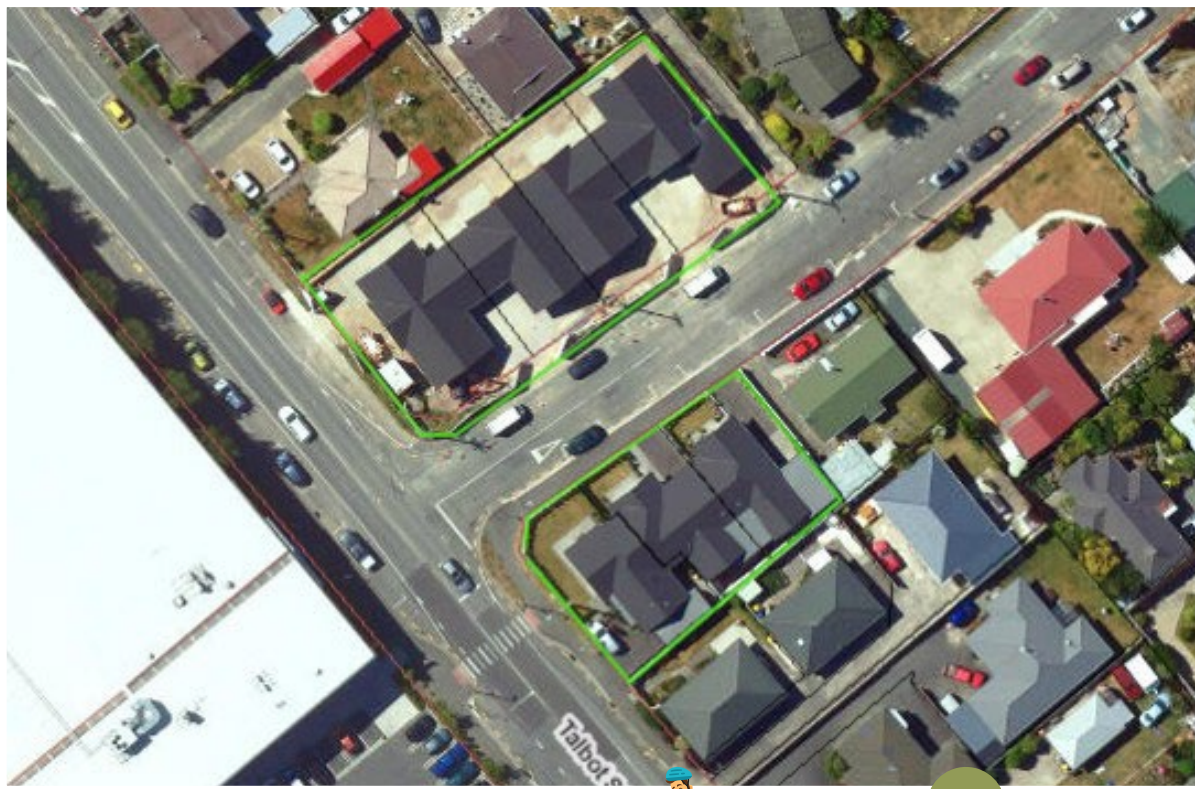
Figure 4. Sections after redevelopment, between three and four single storey attached units on each section, net addition of five dwellings
