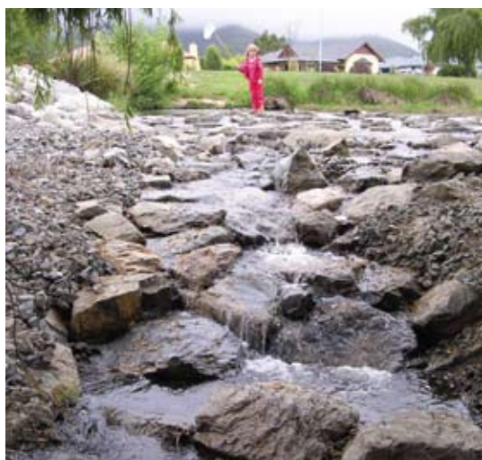
The rock ramp as it is now.
