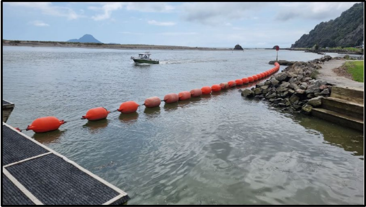
Figure 1: Example of Floating barrier at Whakatane.
