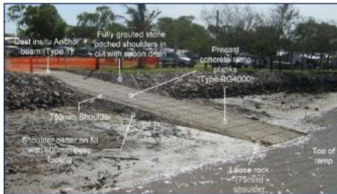
Figure 5: Typical Major Components of a Ramp
