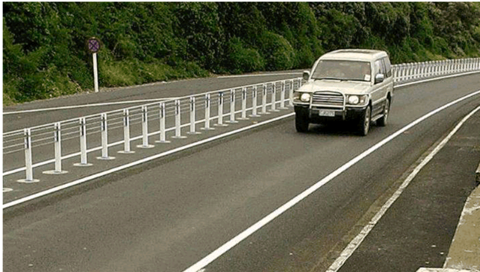
Figure 2: Example of a median barrier
