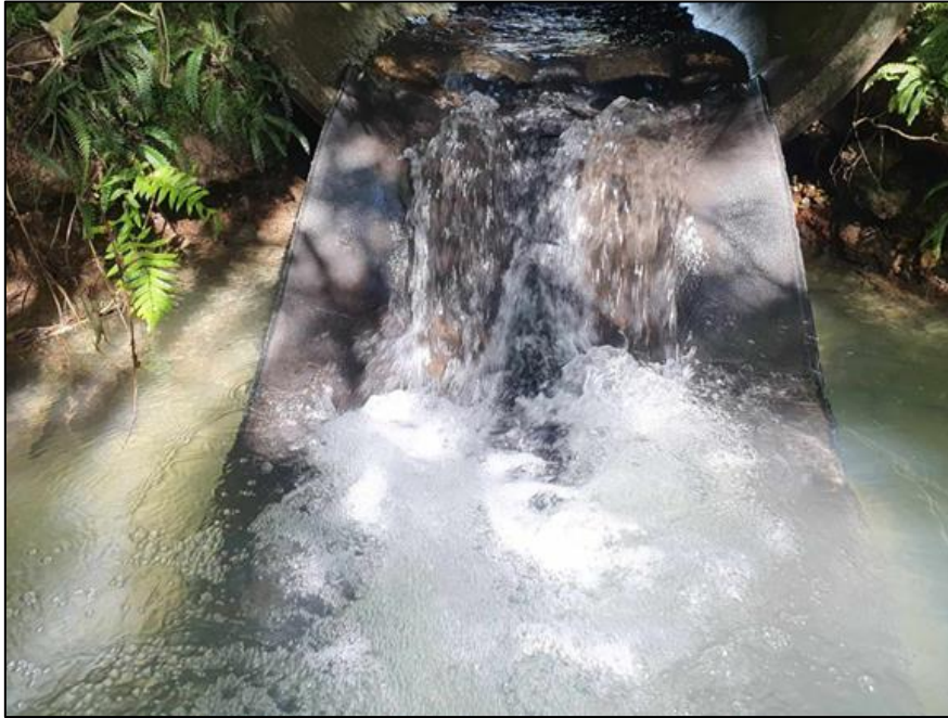
Figure 17. The remediation at Mulligans Creek on the true right culvert, showing a flexible rubber ramp with mussel-rope and a V-baffle.
