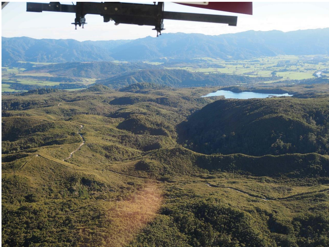
PHOTO 10: Aorere Goldfields Conservation Area, Druggans Dam in distance. The hummocky mined areas generally are in early regrowth scrub, with public trails visible. Limestone areas stand above these. Cave entrances not visible to the right.
