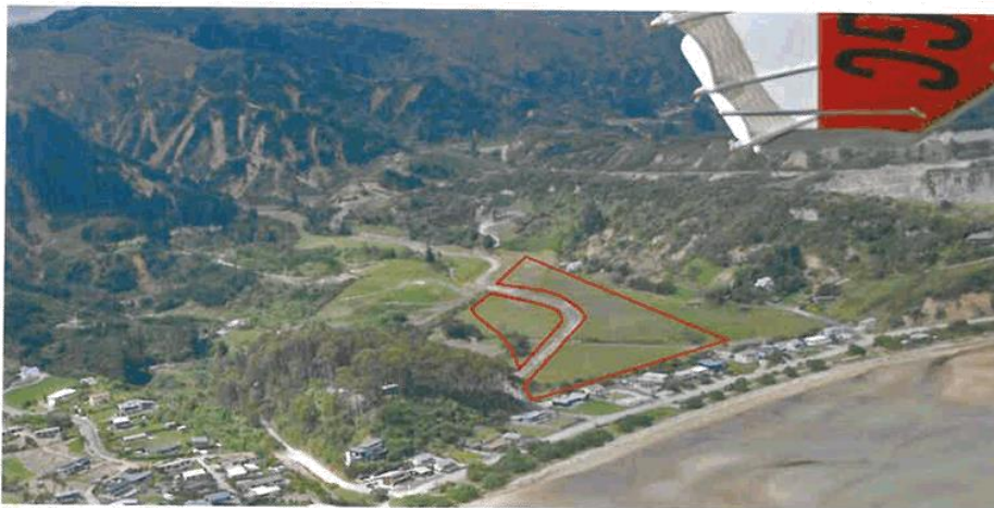
Photograph 4-1: Oblique of the site and hill catchments above showing heavy scarring which generated material that deposited in the lower catchment. Approx. site boundary shown in red. Photo courtesy of TDC.
