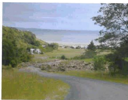
Photograph 4-3: Deposition of debris in channel and on Matenga Road, application site shown beyond.
