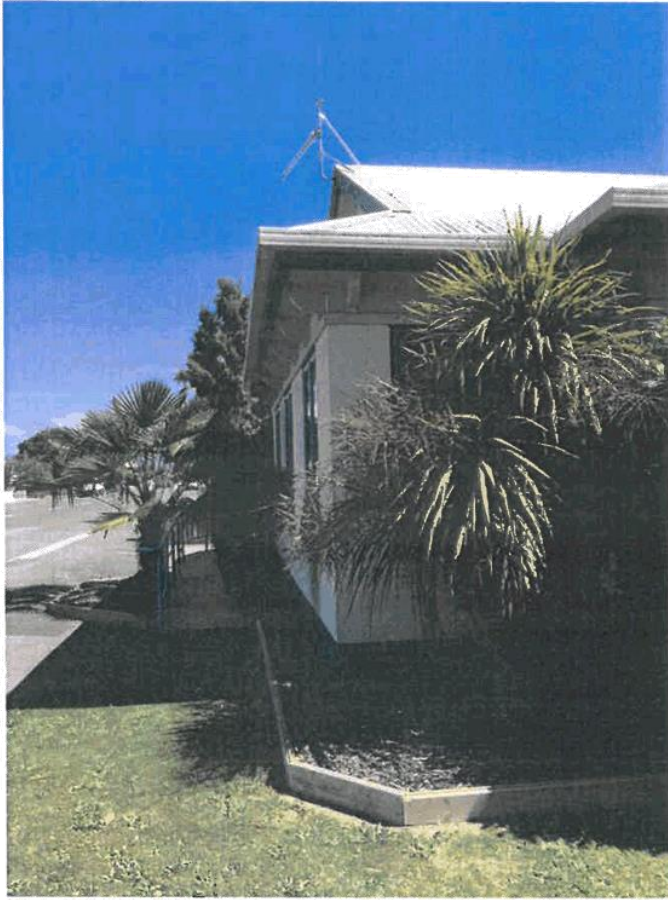
Aerial on roof to look over trees
