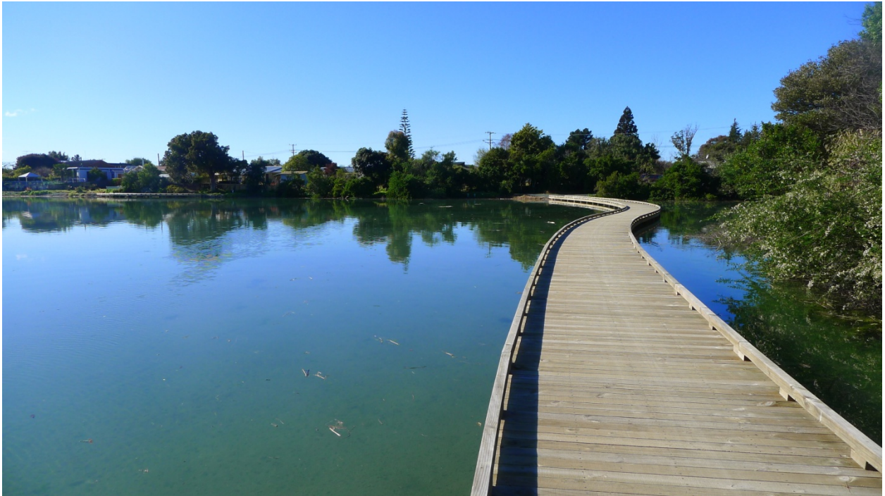
Inlet Walkway, Motueka
