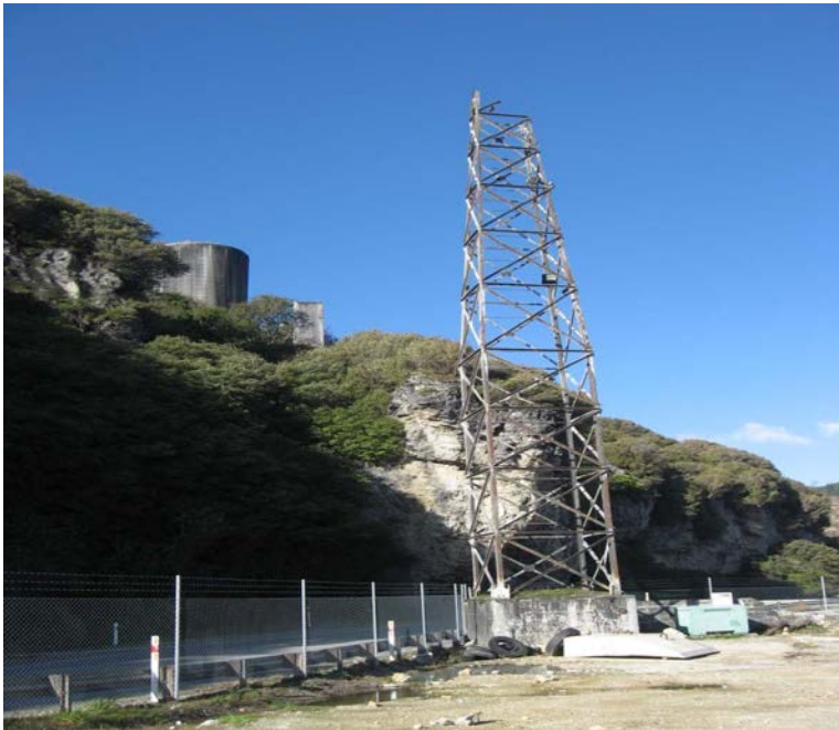
Photograph 19: Old conveyor support tower now used as a light tower
