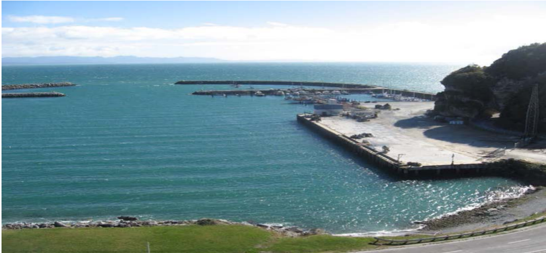
Photograph 1: View of existing wharf and marina area
