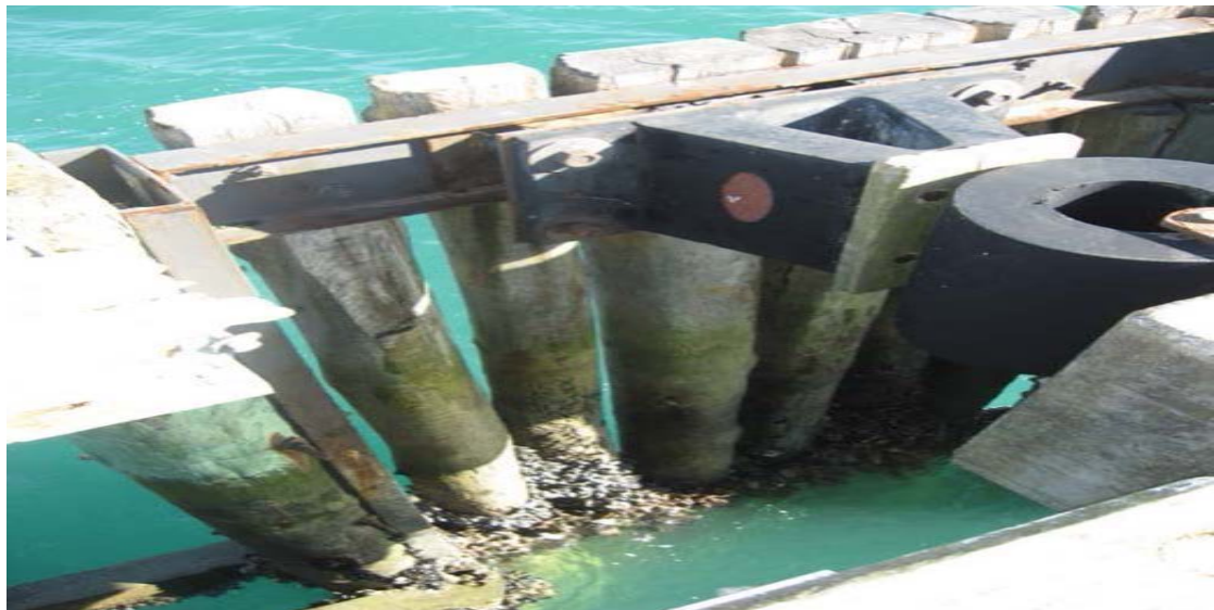
Photograph 5: Showing rubber components of fendered system.
