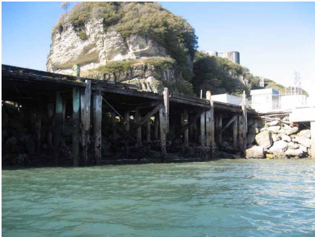
Photograph 13: View of old timber wharf.
