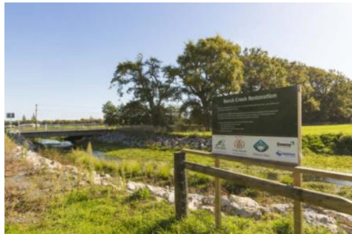
Figure 7 Borck Creek stormwater improvements
