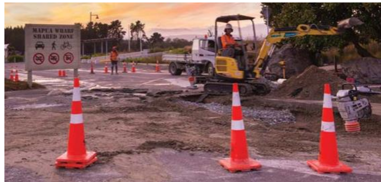
Figure 5 Construction on water and wastewater upgrades in Māpua
