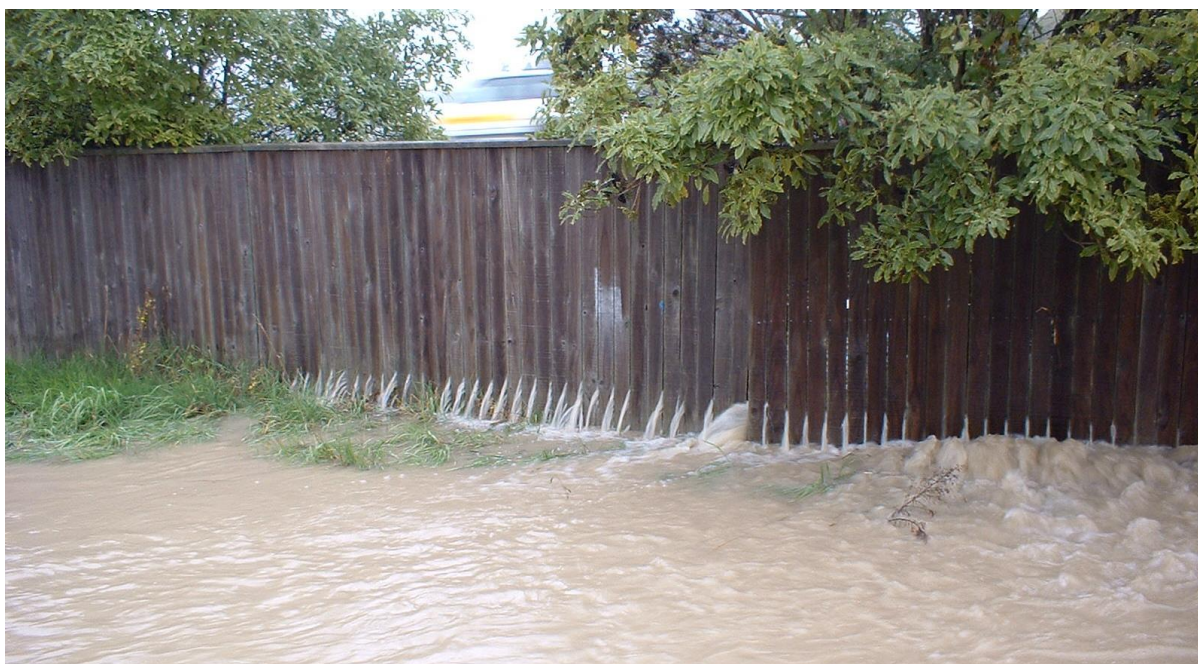
Photograph 2.2: Rintoul Place downstream of 350 mm culvert outlets - August 2022 (source: TDC)
