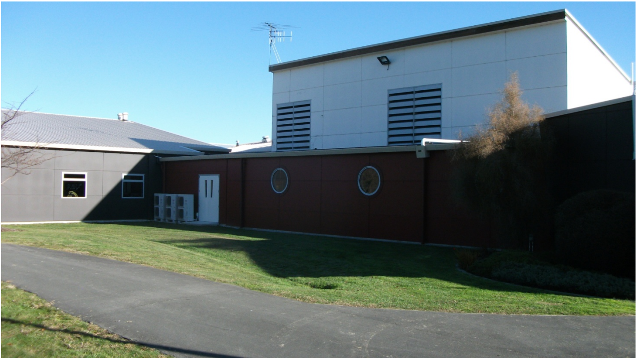
View from North
