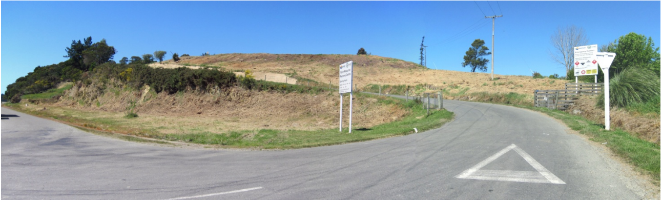
Figure B-7: Mariri RRC – entrance from Robinson Road
