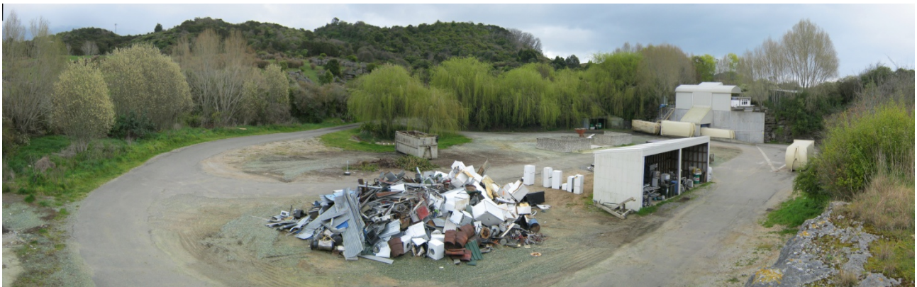
Figure B-10: Takaka RRC – from rear of site, with solid waste compactor and bins in background
