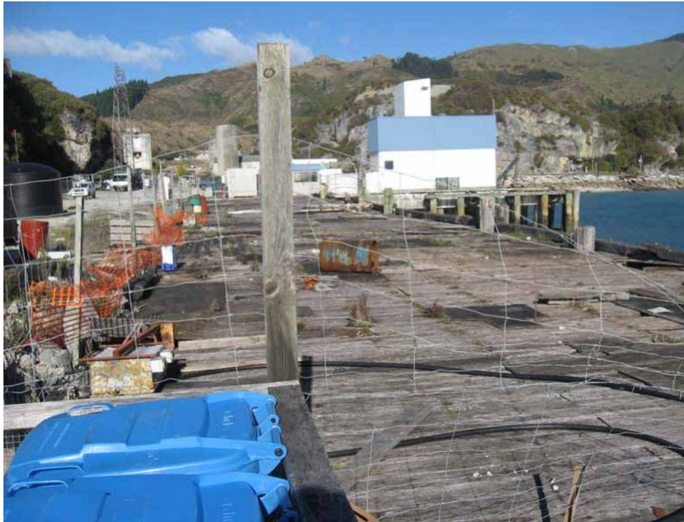
Photograph14: View of deck of timber wharf (condemned and retained for future development).
