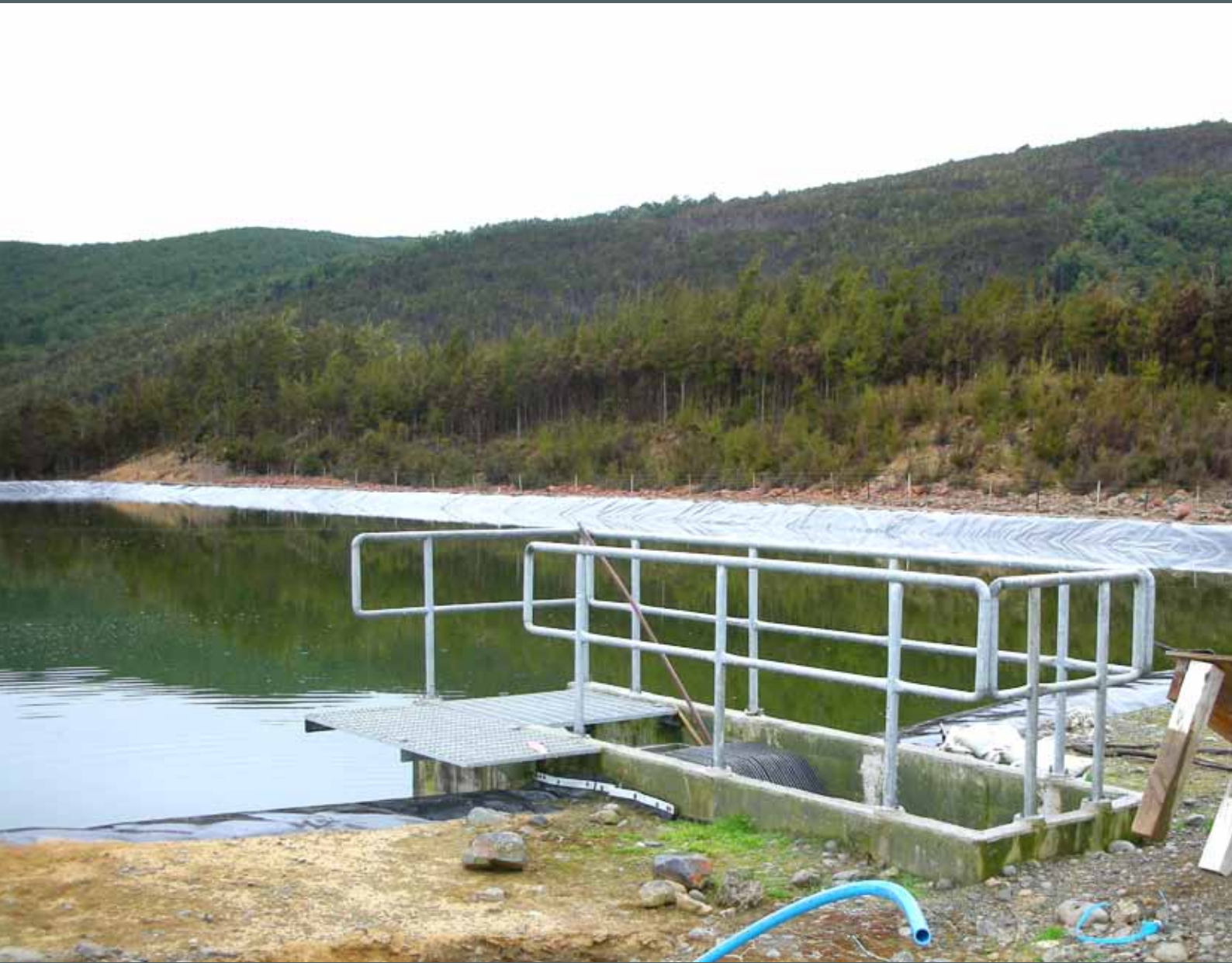
St Arnaud wastewater treatment plant
