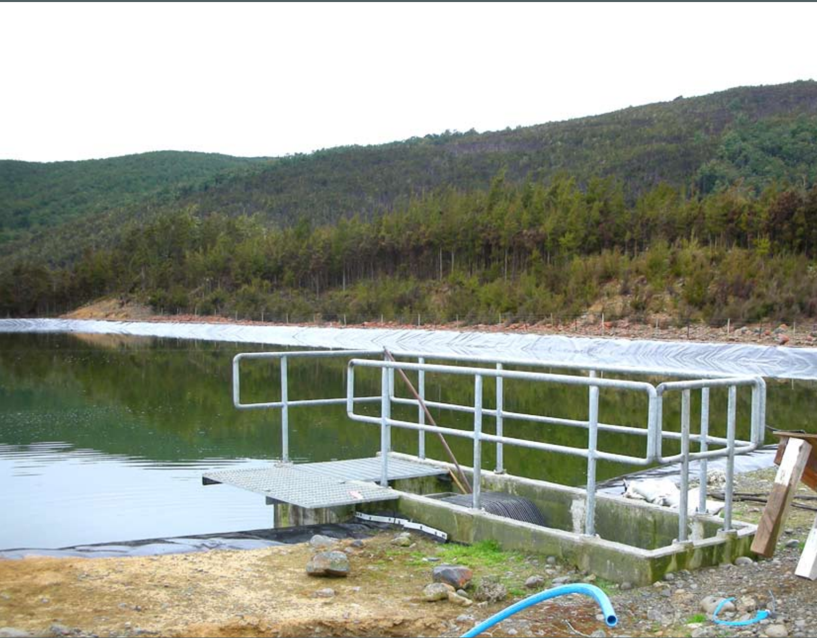
St Arnaud wastewater treatment plant.
