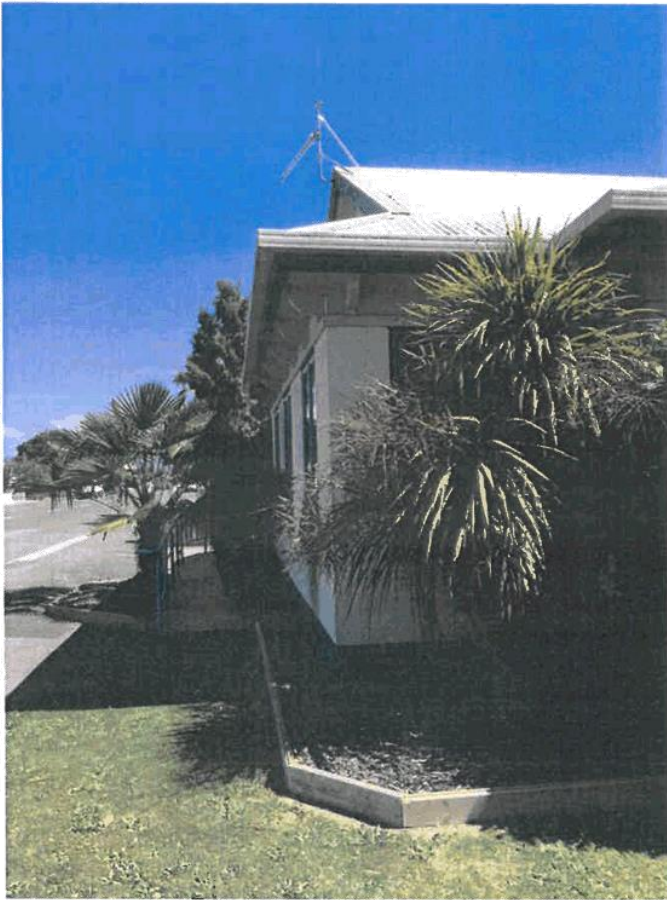
Aerial on roof to look over trees
