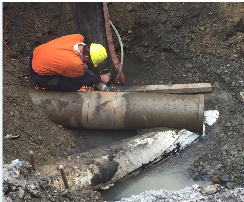
Removal of steel casing penetrating watermain in Lower Queen Street
