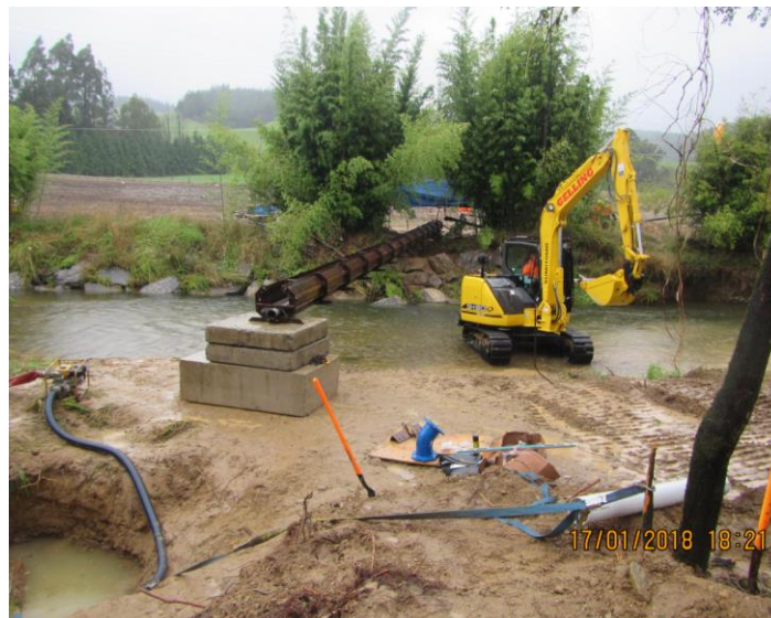
Temporary pipe bridge across Dove River
