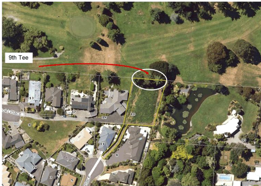
Aerial image 2: Showing potential flight of a sliced drive off the 9 th tree and the screening role of trees to neighbouring property
