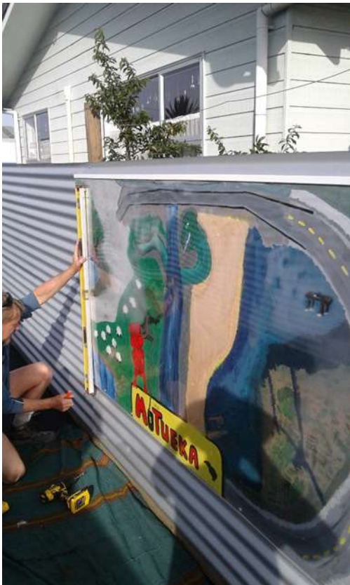
INSTALLING - YMCA MOTUEKA ART PANEL
