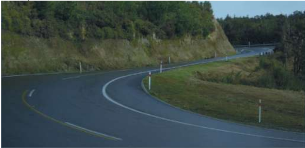
SH6 Hope Saddle approaching from the North
