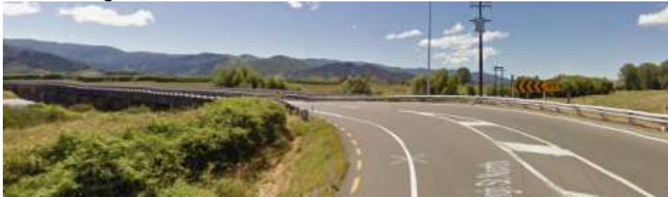
SH60 Motueka Bridge approaching from Motueka
