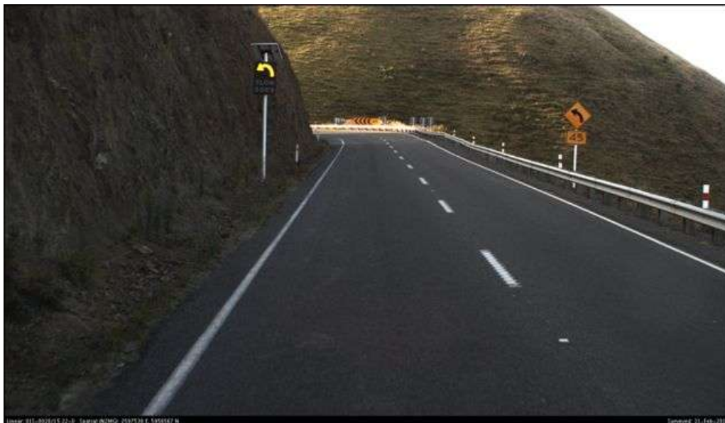
Weld Pass SH1 south
