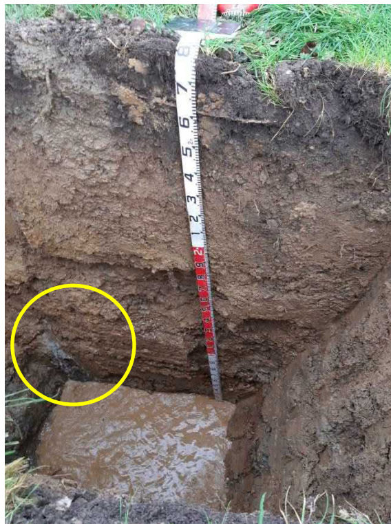
Figure 10. Groundwater at Test Pit TP07 showing spring in side wall
