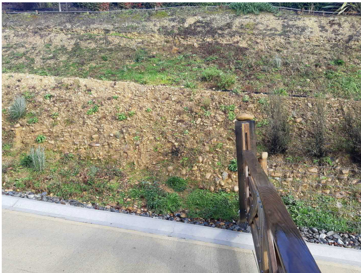
Figure 9. Slope at 52 Cupola Crescent Accessway
