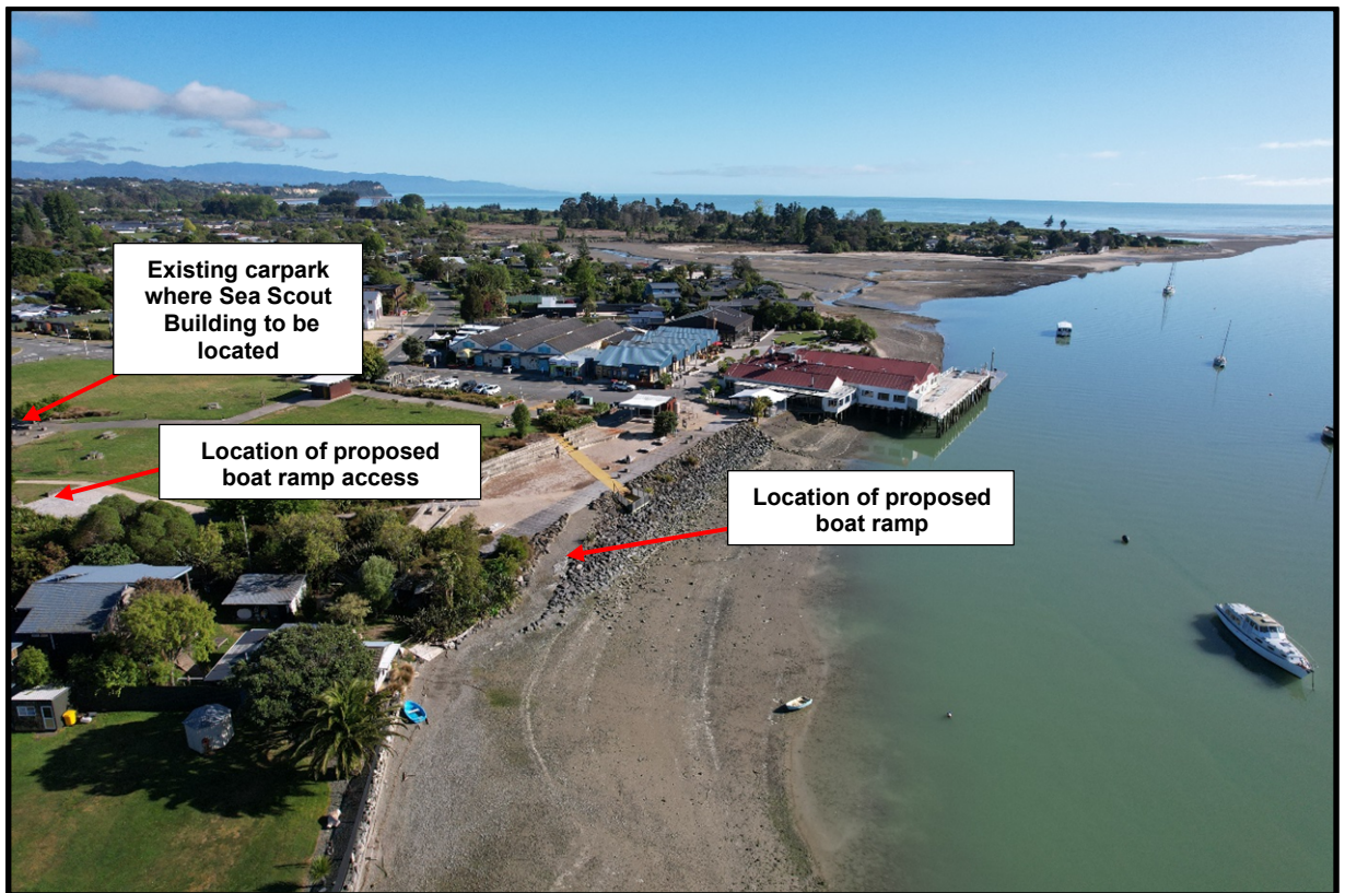
Figure 1: View of the proposed boat ramp site.
