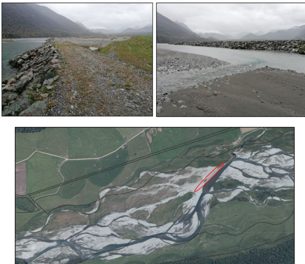
Figure 2.7: The construction of a 200m long rock wall on the Matakītiki River downstream of Mole Stream in 2020 has the potential to reduce the number of active river braids and gravel islands within this regionally important site for coastal birds. The red circle in the aerial photograph shows the location of the rock wall, demonstrating how it acts to confine the majority of the river flow to the main channel and prevents water from travelling through a series of braids on the true right of the channel. Image Credit: Trevor James/Tasman District Council.
