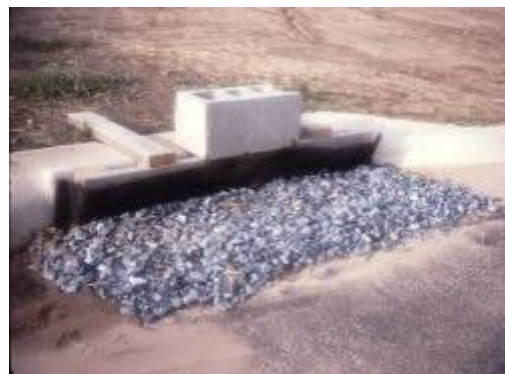
Figure 9-25 Inlet protection with aggregate on top of geotextile fabric
