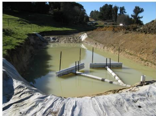
Figure 9-1 Sediment Retention Ponds (forebay in foreground of upper photo, decants in lower photo)
