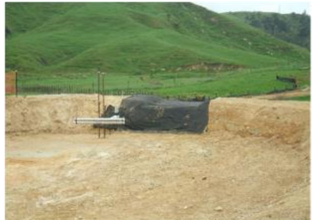
Figure 9-16 Decanting Earth Bund
