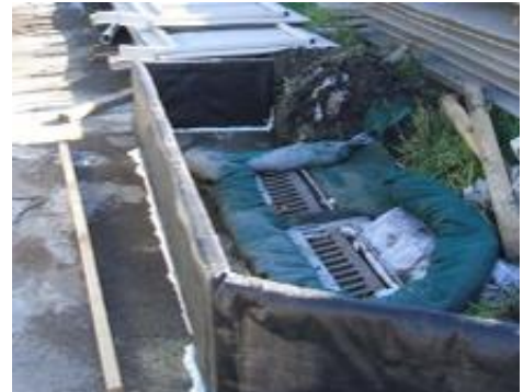
Figure 9-24 Stormwater Inlet Protection – silt fence and geotextile sock
