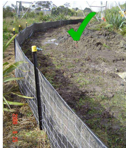
Figure 9-14 Super Silt Fence
