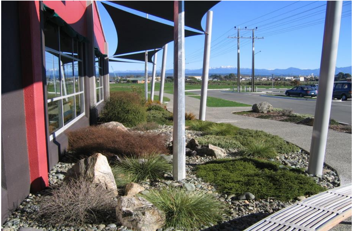
Figure 1: Richmond Aquatic Centre frontage.
