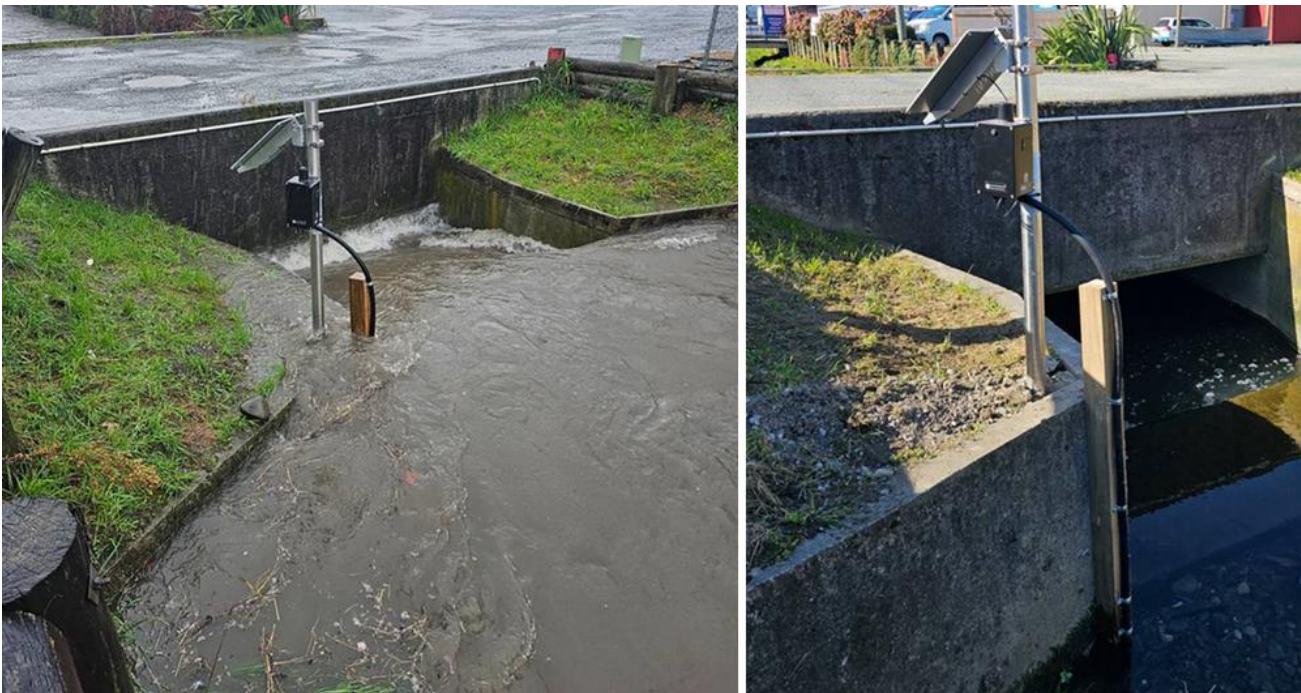
Figure 2 Beach Rd continuous monitoring site
