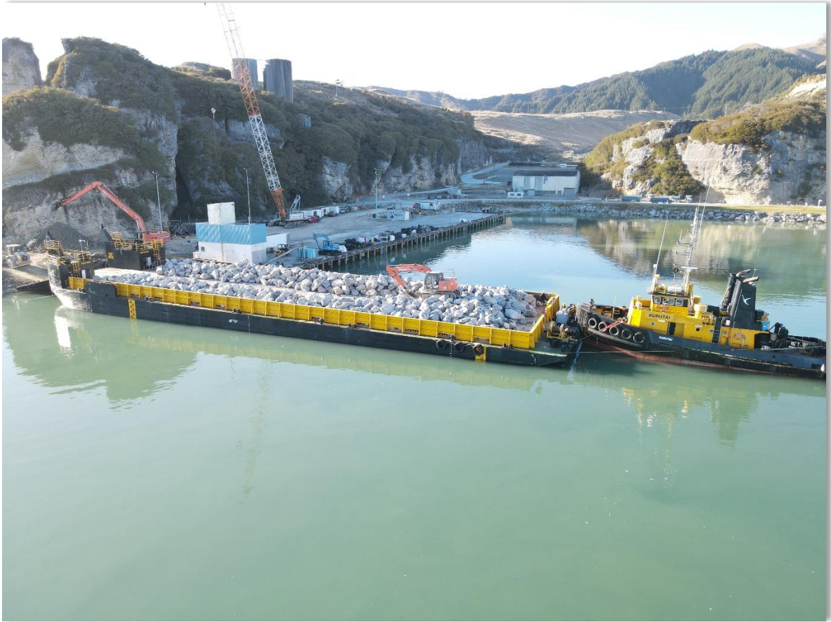
Figure 2 Rock loading onto barge
