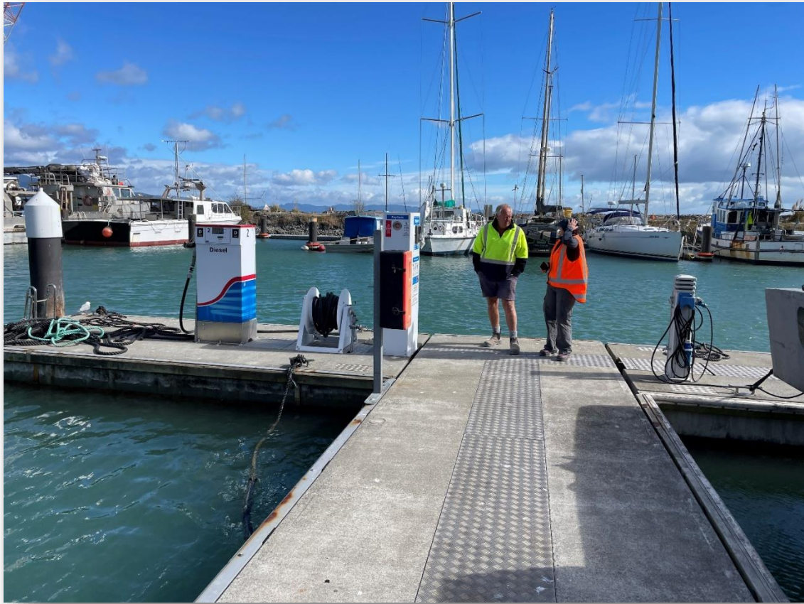
Figure 4 Fuel bowser on floating dock.
