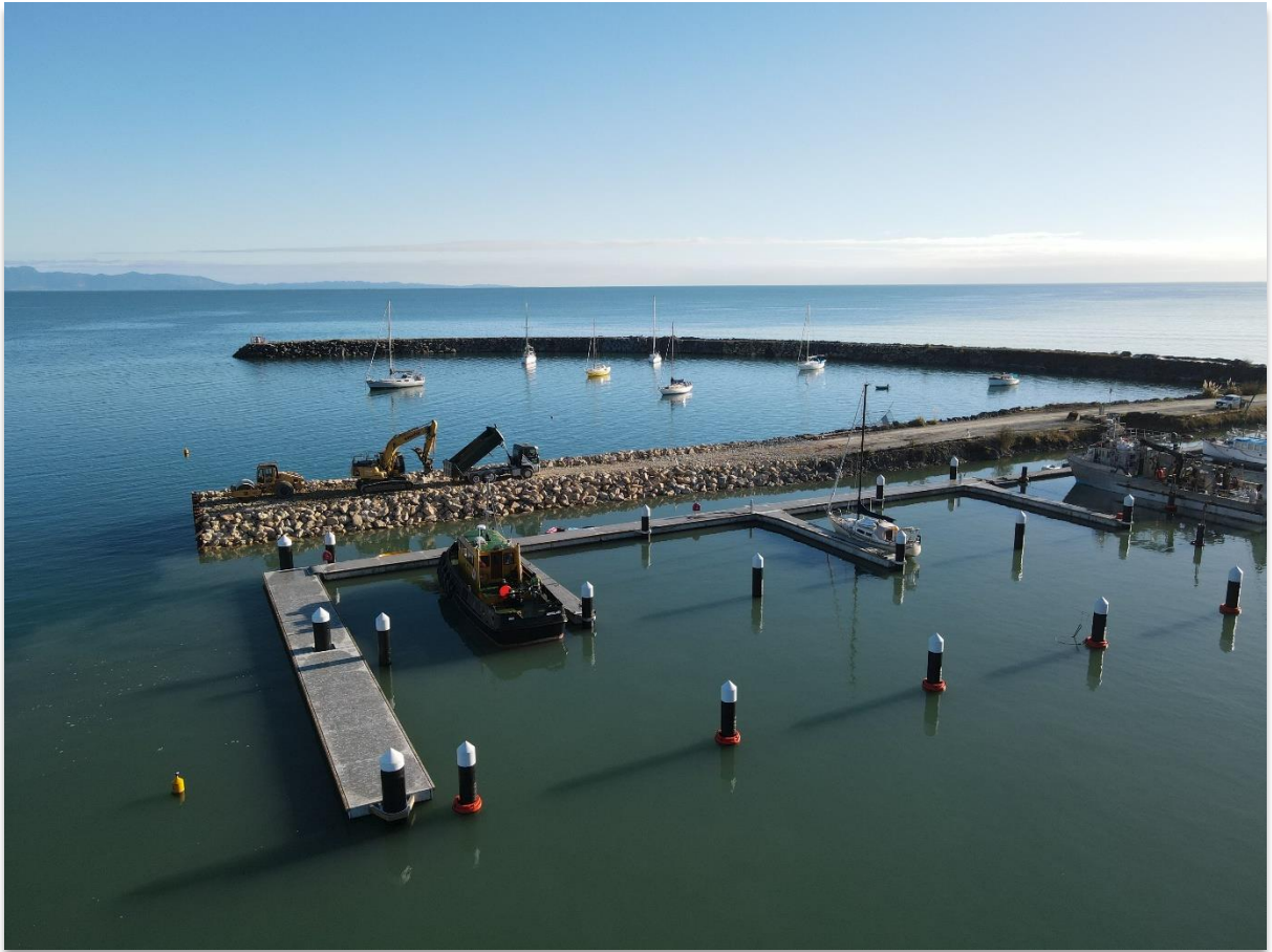
Figure 3 New berths with floating concrete platforms
