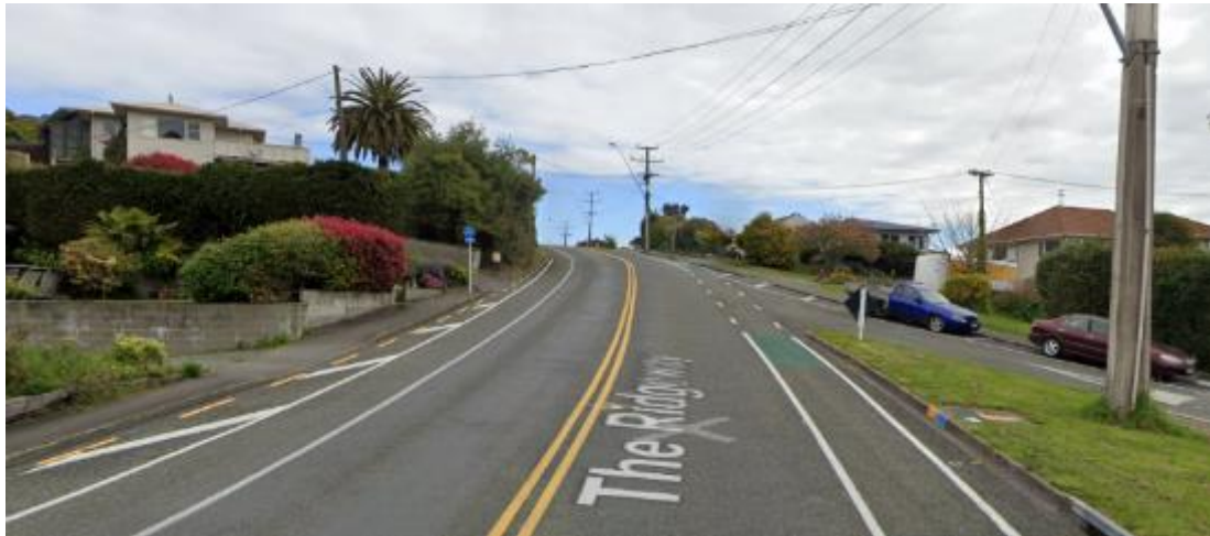
The Ridgeway SAAS: 40km/h (50 with separated cycles) Current Limit: 50km/h Mean Speed: 46km/h
