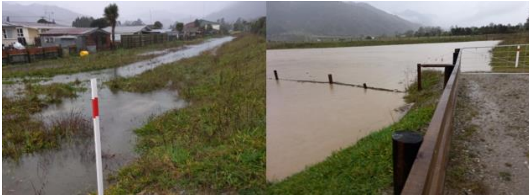
Minor ponding between backs of properties, north of new stop bank (L) and flooding in new ponding area south of stop bank (R) – Hampden Street, Murchison.
