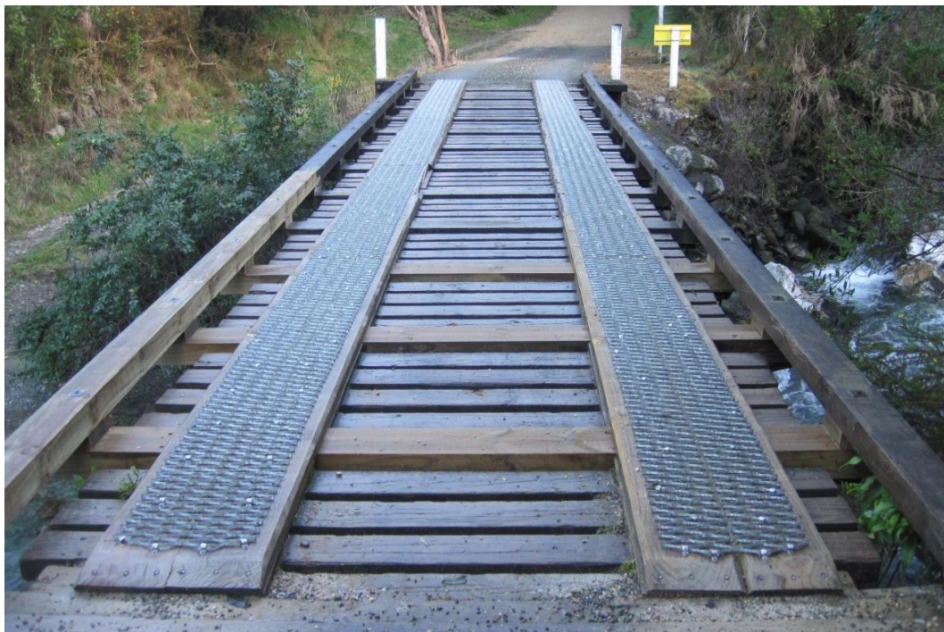
Walsh Creek bridge repair
