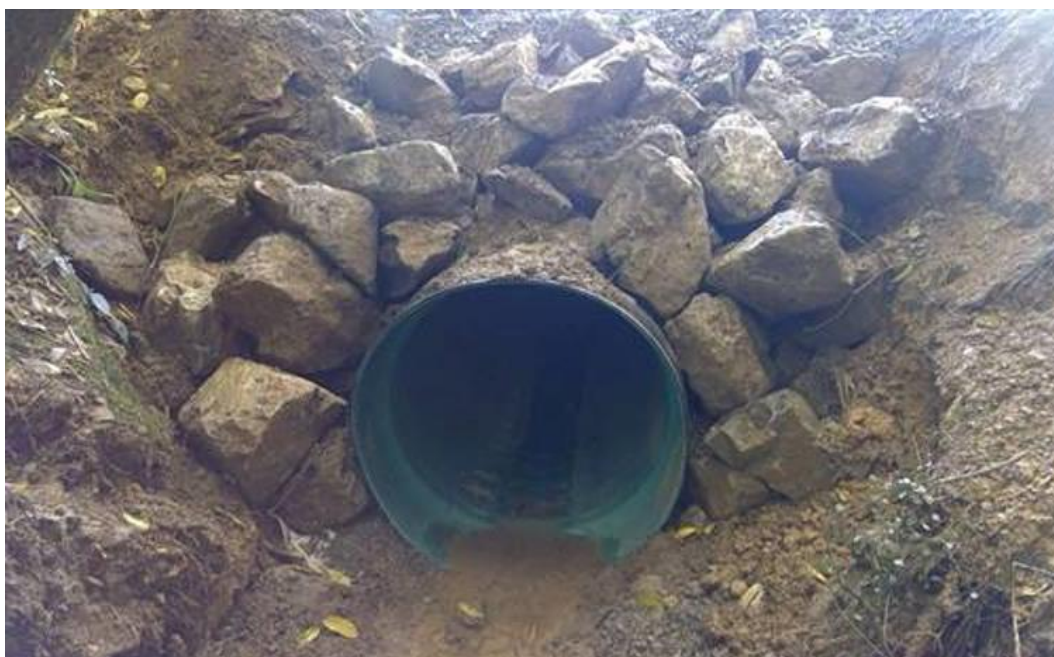
Replacement culvert Rosedale Road
