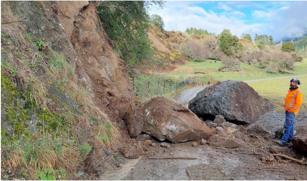
Glenroy Road slip
