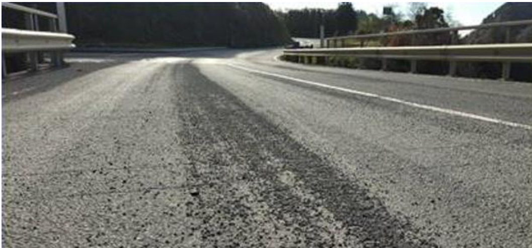
Gritting – Wairoa Bridge
