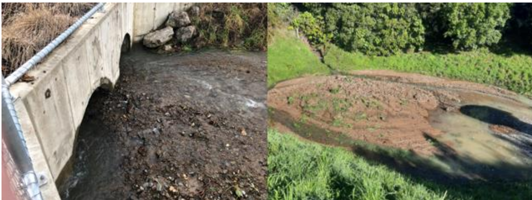
Accumulation of gravels – Pine Crest Drive twin culvert outlet, Richmond (L) and Lodestone Detention Dam, Richmond (R)
