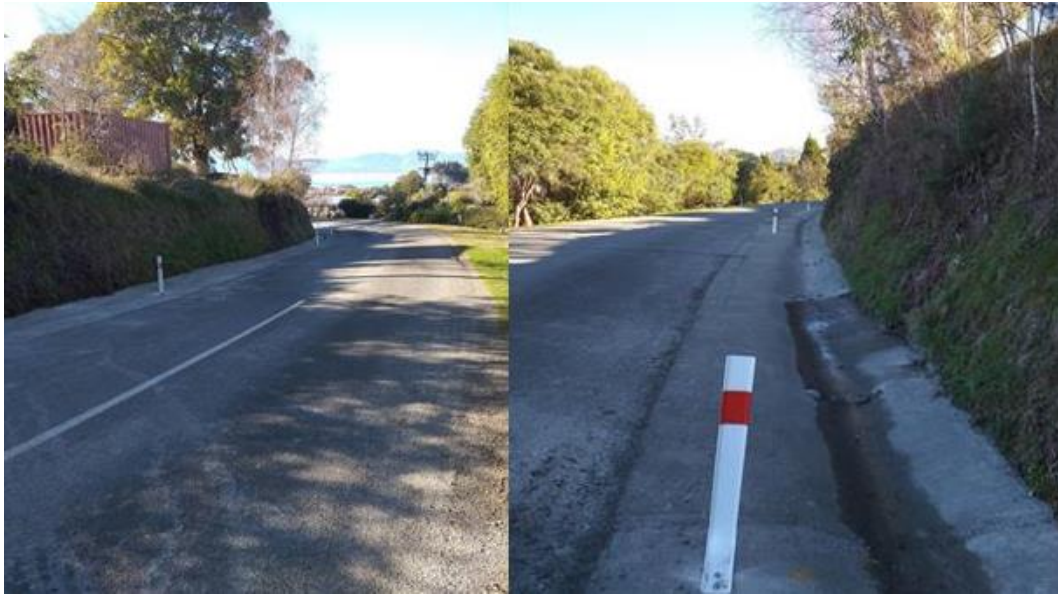
Pomona Road – new concrete swale
