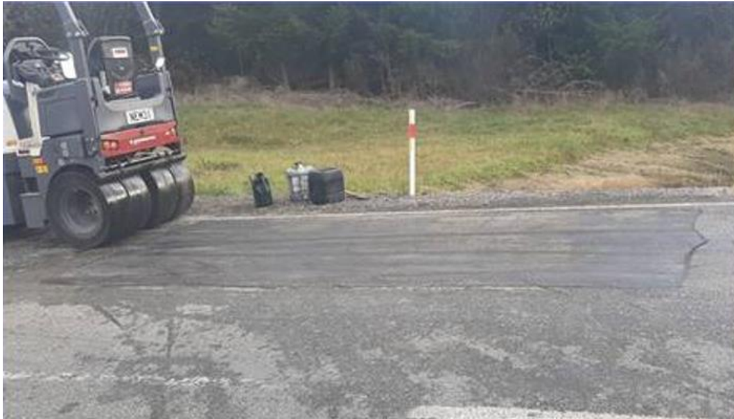
AC repairs underway
