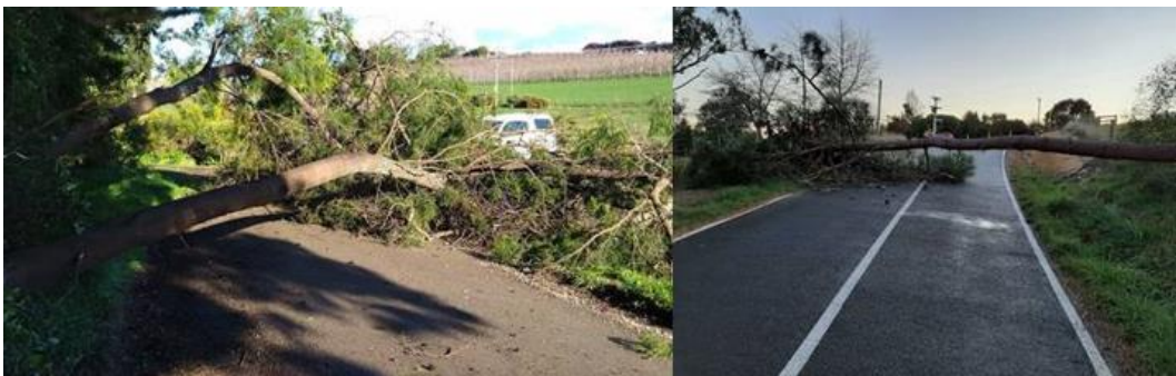
Various trees down requiring clearing
