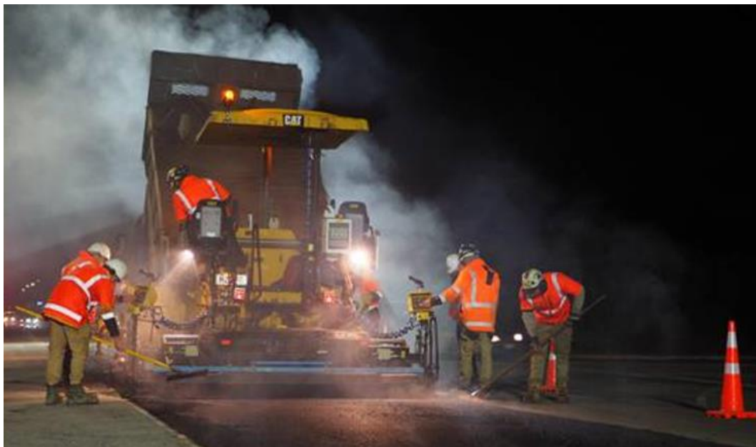
AC renewal work on Berryfields/McShane Road
