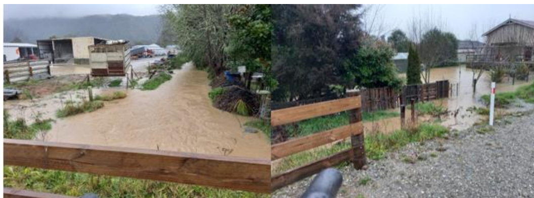
Flows below flood detention area transport yard (L) and property on Hampden Street (R).
