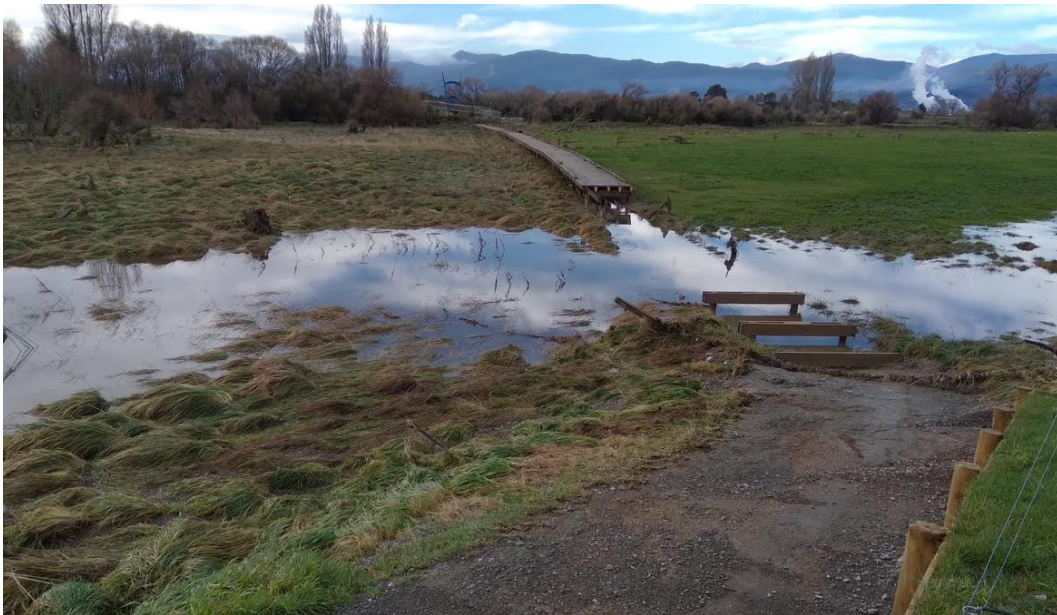
Flood damage to cycle trail boardwalk, Waimea River
