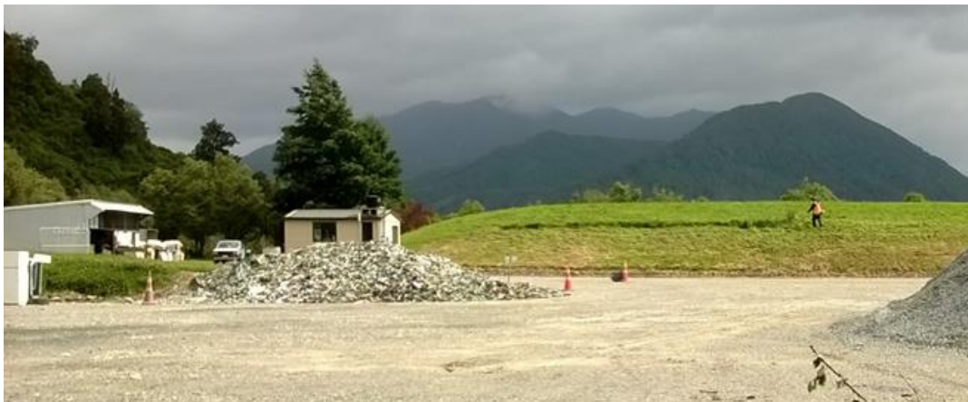
Figure 9: Murchison RRC – Recycling Shed on Left Background and Closed Landfill to the Right
