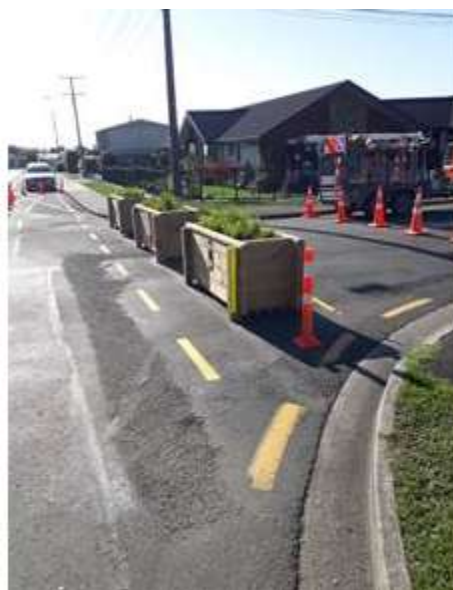
Elizabeth St/Talbot St intersection
