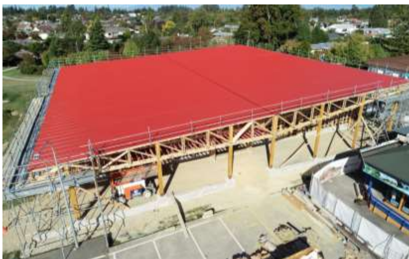
Roof close to completion, 22 March
