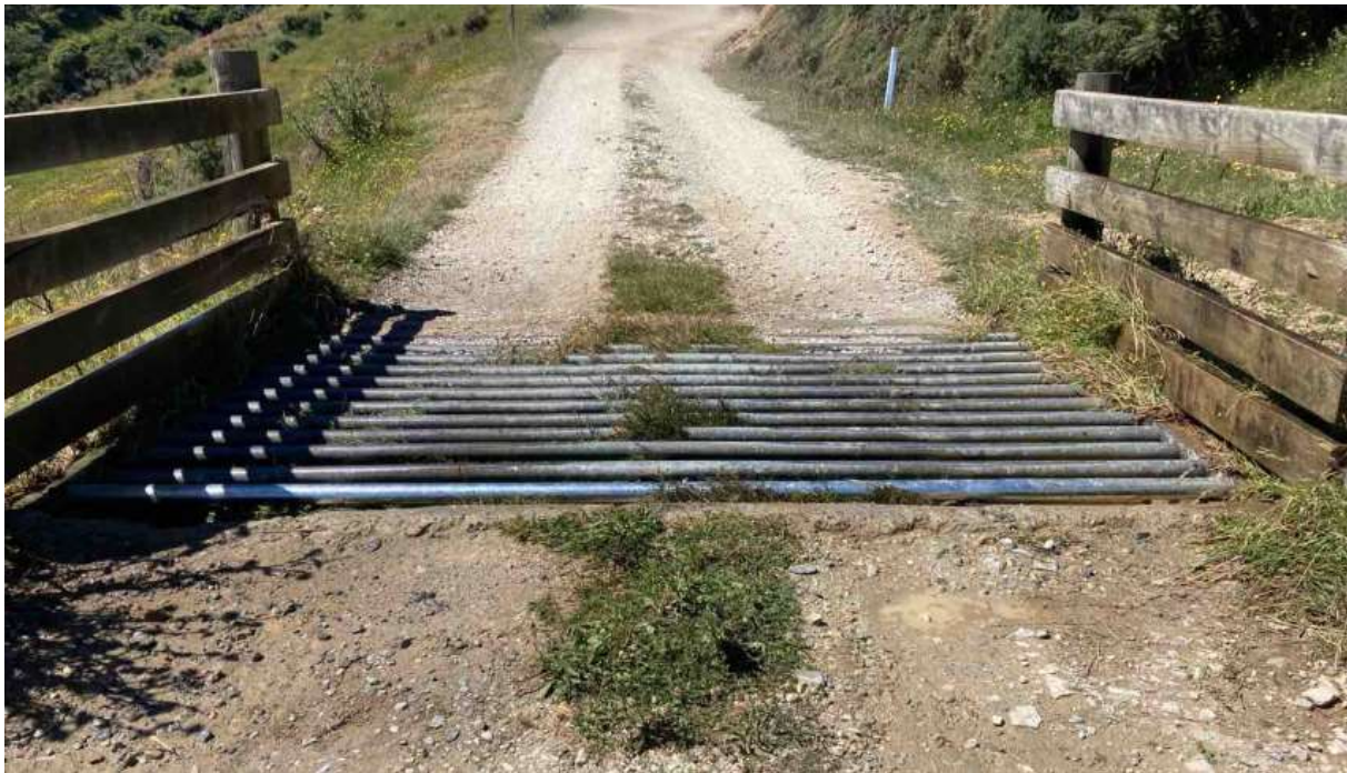
Limestone Road cattle stop repair
