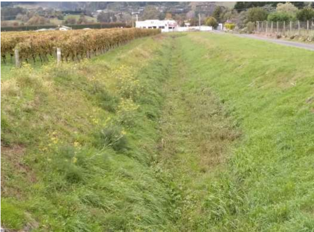
Upper Borck Creek downstream from State Highway 6, Hope
