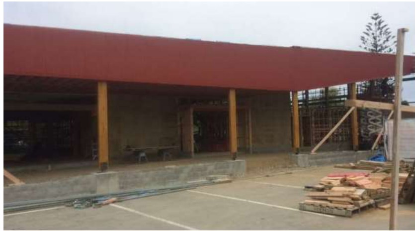
Roof facade completed, 20 April
