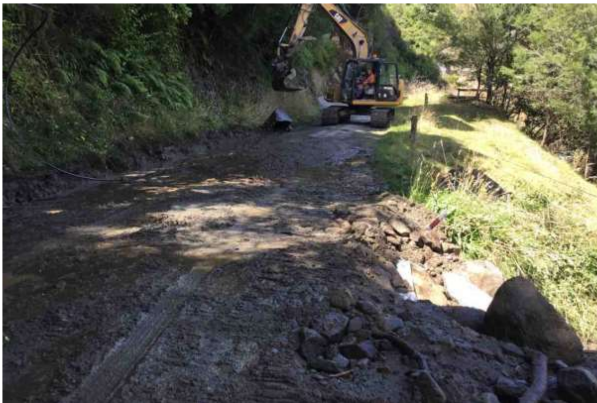
Glenroy washout repair
