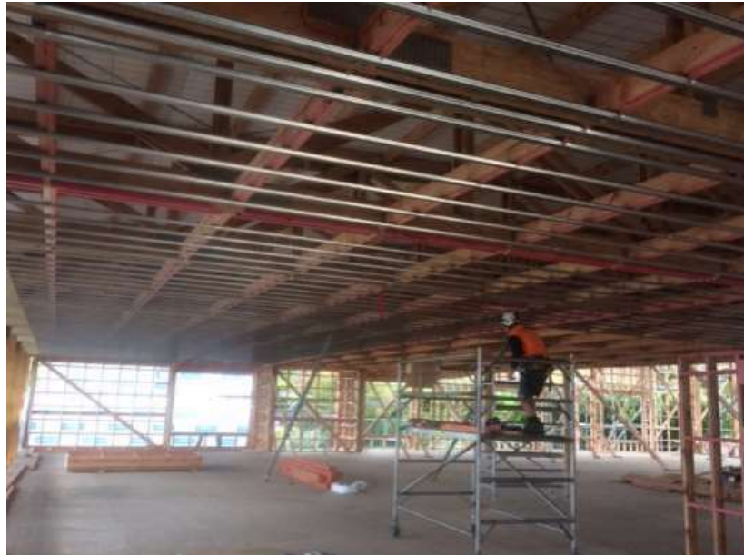
Fitting of supports for the ceiling diaphragm, 20 April
