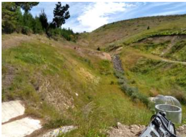
Two new detention dams at Katania Heights, Brightwater
