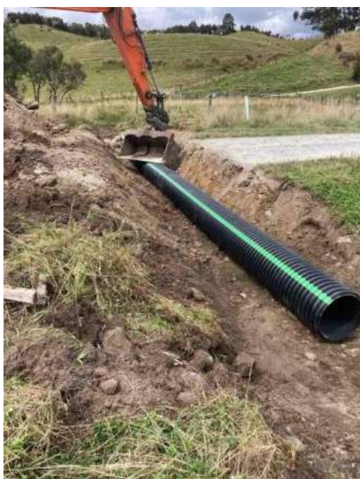
Quartz Range Road – culvert replacement with farm boss pipes
