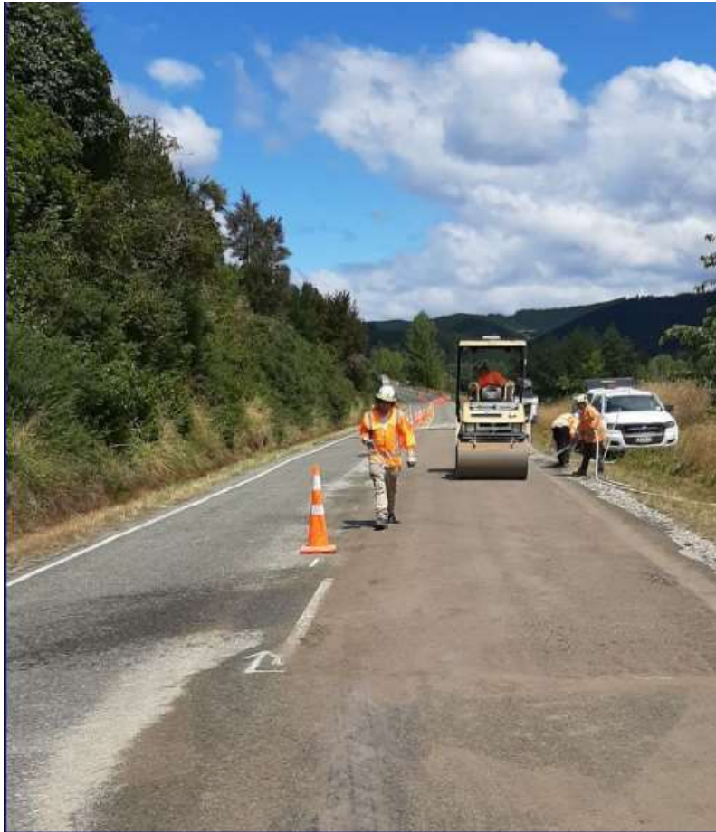
Emulsion stabilising sealing – Wai-iti Valley
