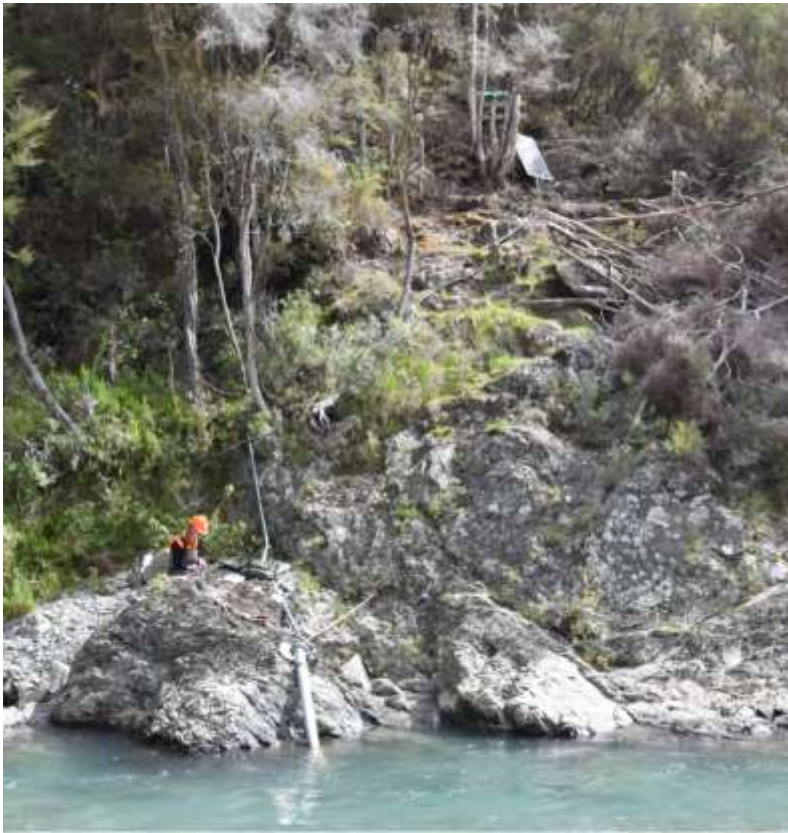
Figure 3 – Turbidity monitoring site downstream of WCD construction site
