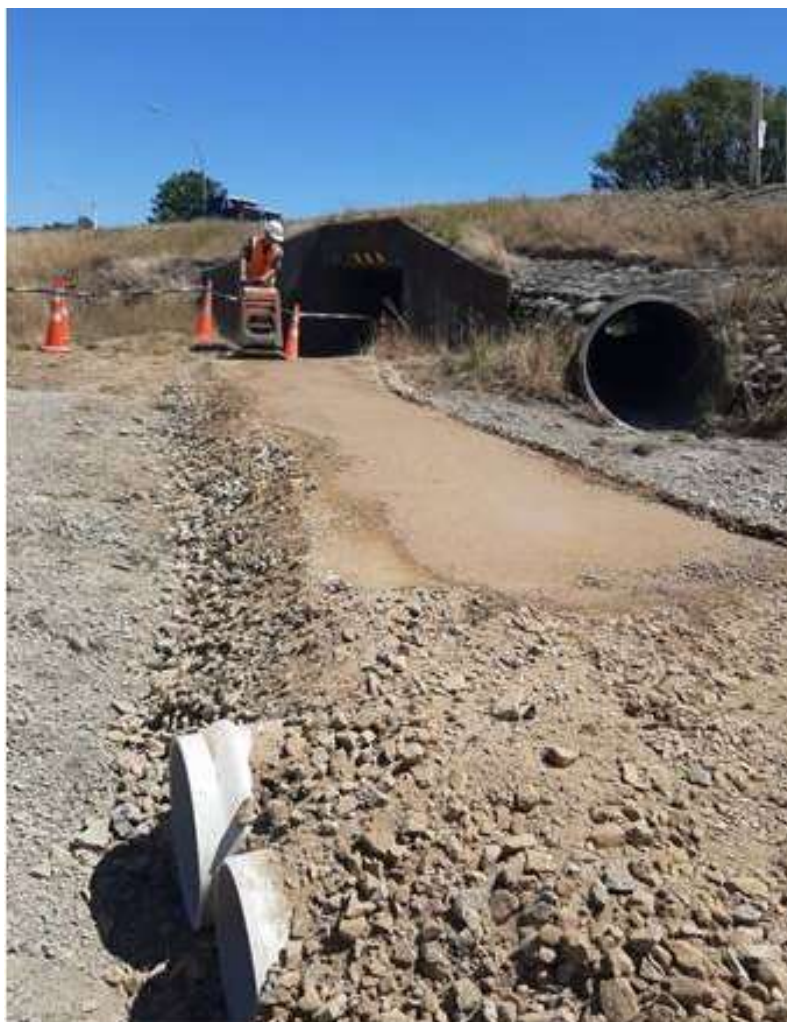
Brightwater underpass raised footpath
