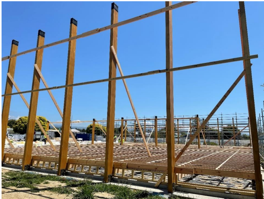
7 Support columns in place ready for installation of flooring
