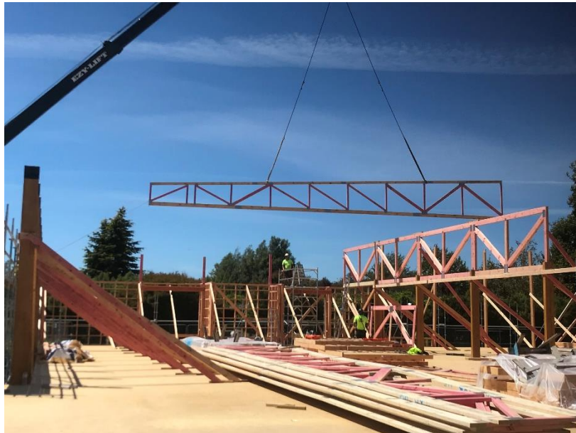
10 11 Installation of roof trusses
