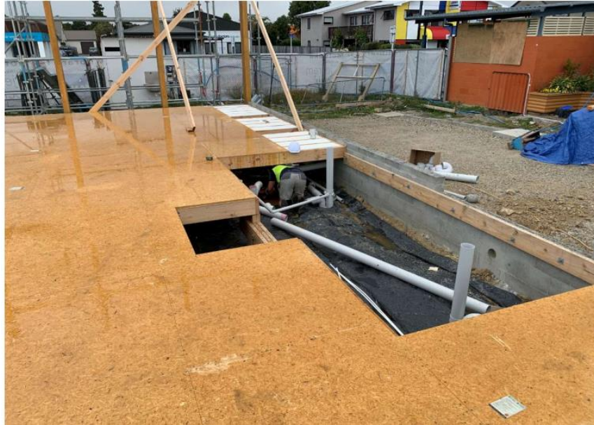
8 9 Floor installation underway – public toilets and i-site to the right
