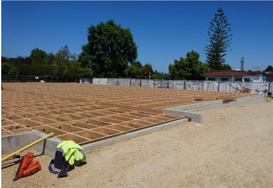
5 Floor joists in place – looking towards Wallace Street
