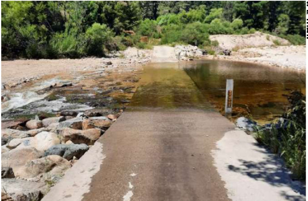
Figure 3. Dart Ford current state. Note the rock ramp/apron on the downstream (left) side that will act to prevent cars from being swept away in higher flows.
