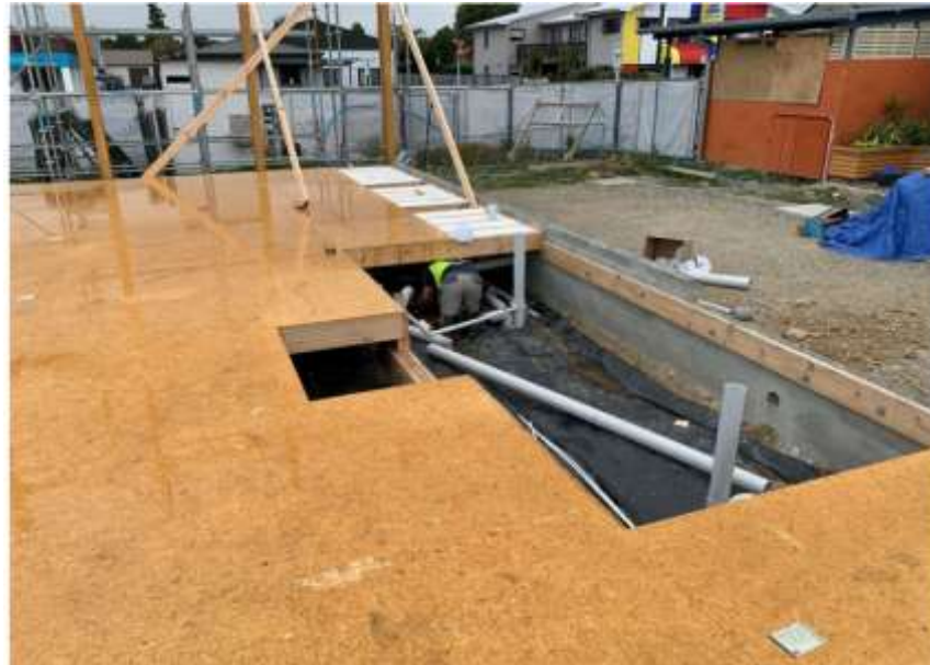
Floor installation underway – public toilets and i-site to the right
