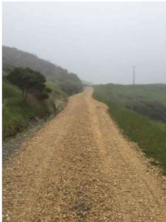
Limestone Road metalling
