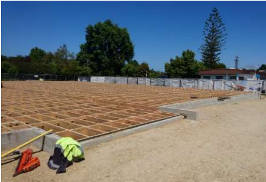
Floor joists in place – looking towards Wallace Street
