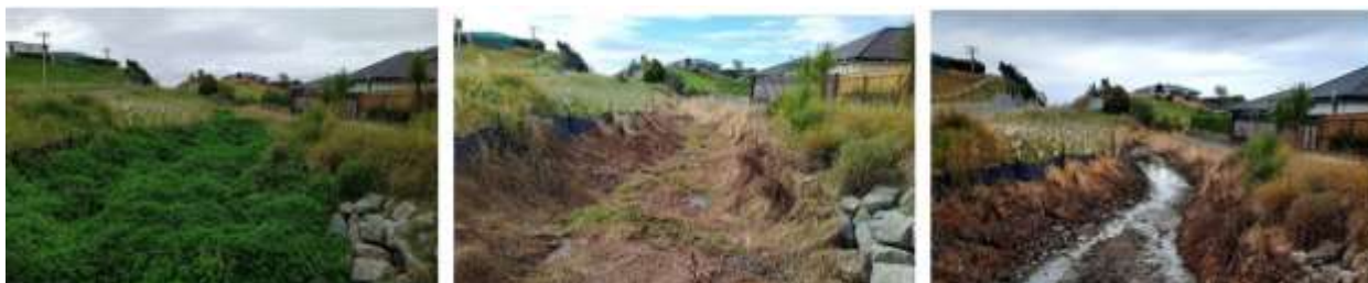
Spray control of Vietnamese Parsley and Water Celery – Eastern Hills Drain, Hart Road, Richmond – before (L) after (C), and after raking out (R).
