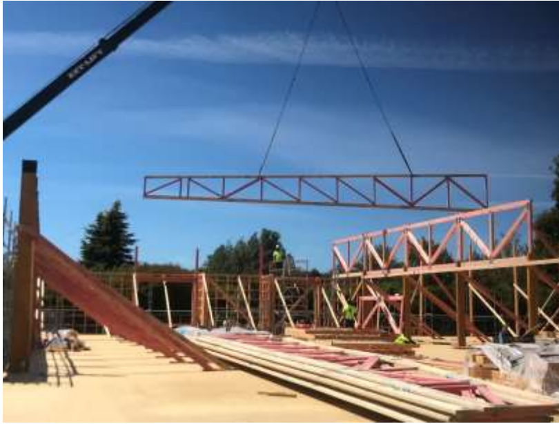
Installation of roof trusses
