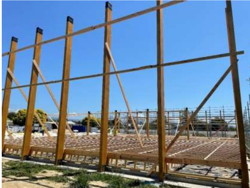
Support columns in place ready for installation of flooring
