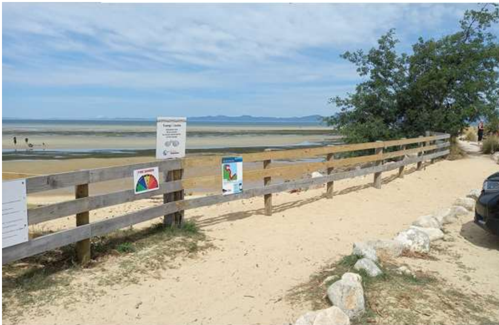
Sandy Bay-Marahau Road Footpath and Fence Repairs
