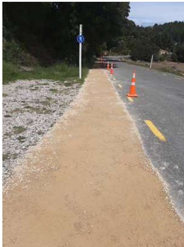
Martin Farm Road footpath maintenance
