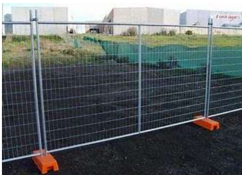
Figure 1: Temporary site fencing.
