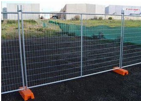
Figure 1: Temporary site fencing.
