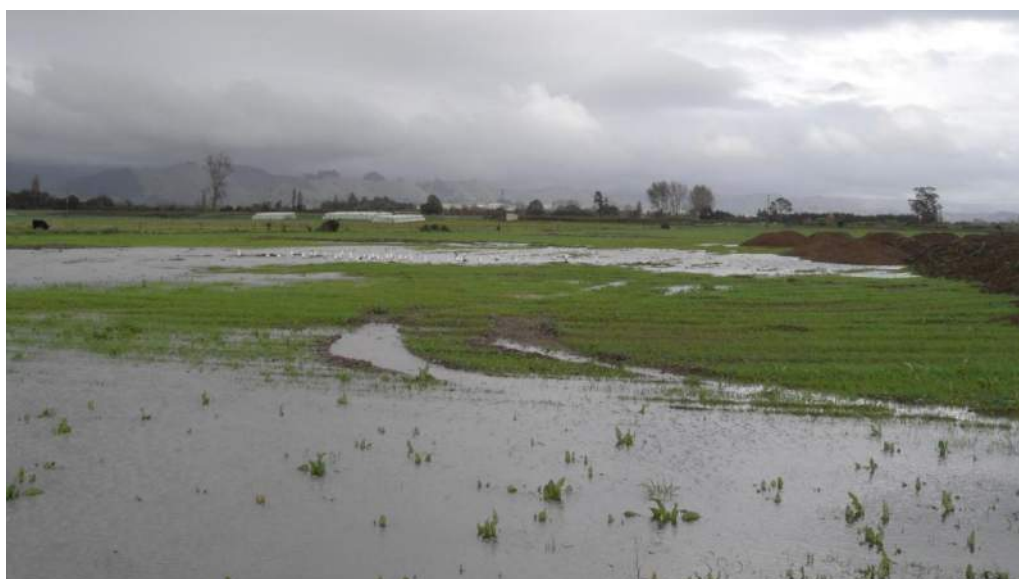
Figure 13. Water ponding on restored land.
