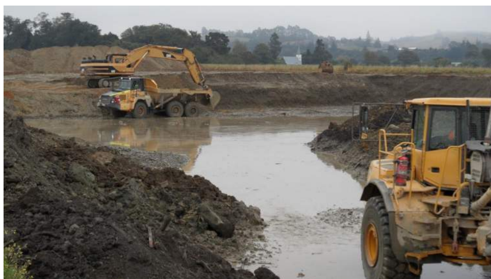
Figure 14. Excavation and backfilling.
