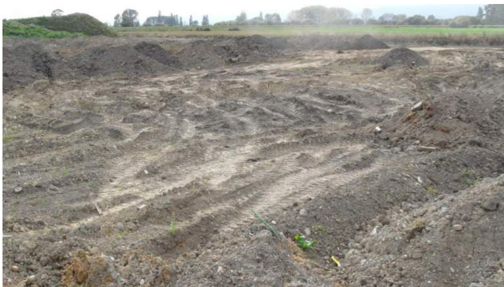
Figure 20. Earth spreading and compaction.
