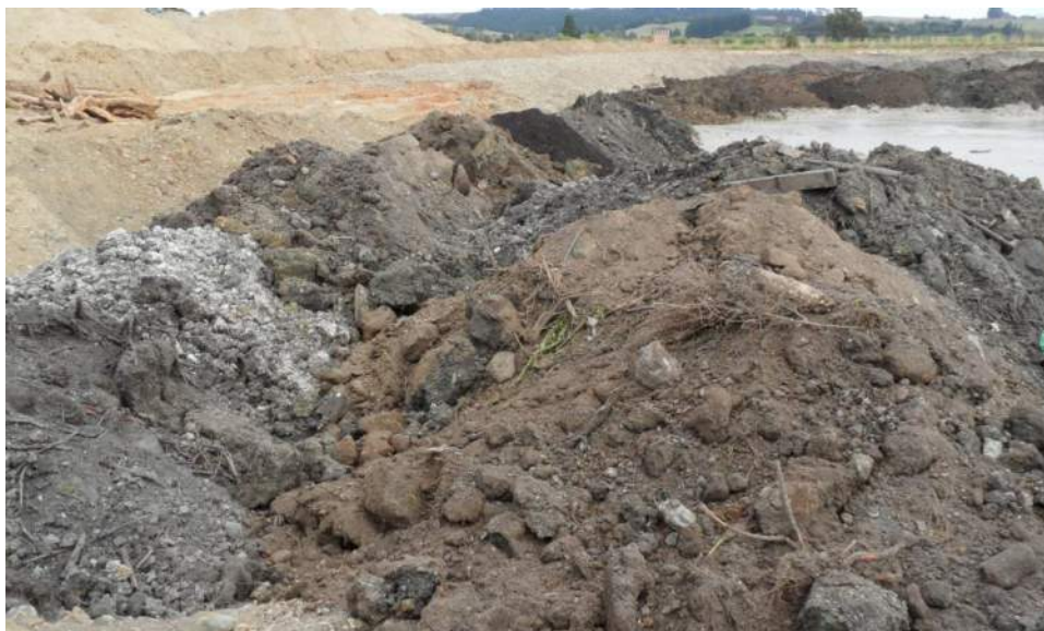
Figure 15. Backfill showing the variety of materials being deposited.
