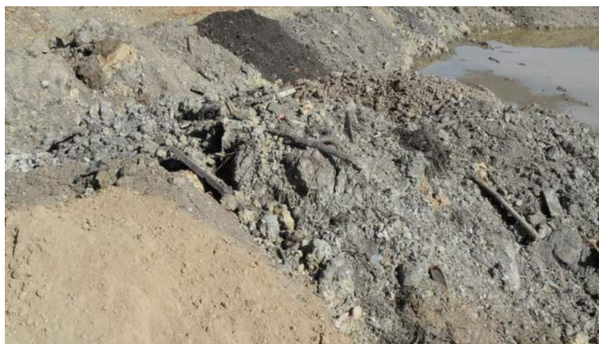
Figure 16. Backfill showing materials being deposited.
