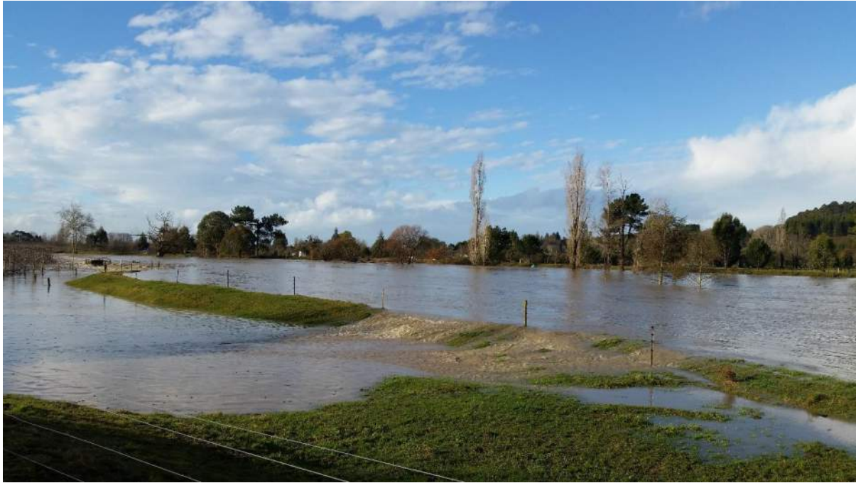
17 July 2021 - Stage 1 site in peak flood.
