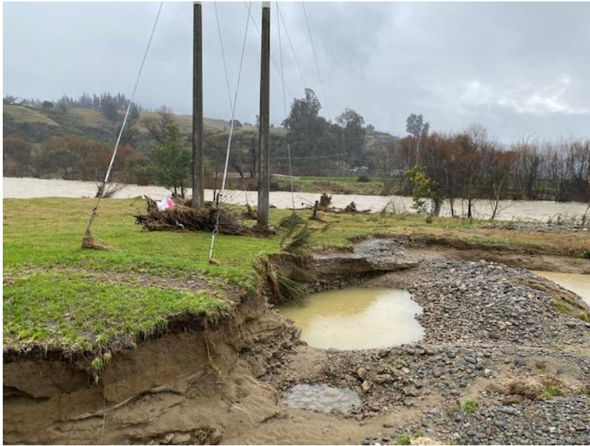
Figure 6. View west of headcut erosion of fine-grained floodplain sediments at the upstream end of the northern pit at Douglas Road following the 17-18 July 2021 flood. The Motueka River is in the background. (Photo provided by Pete Taia)
