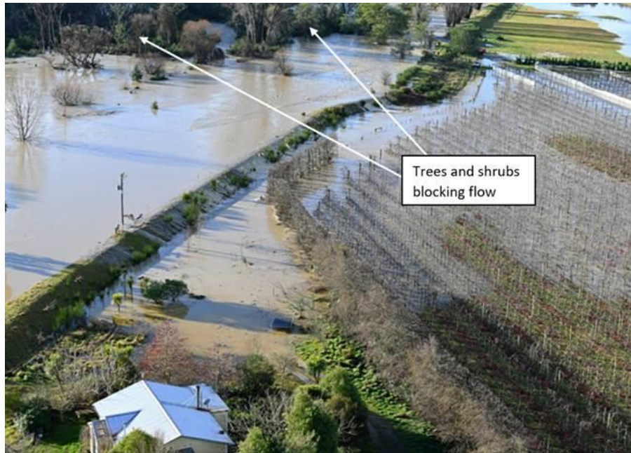
Figure 3. Overtopping of the west Peach Island stopbank during the July 2021 flood. The backchannel is located to the left of the stopbank. (Photo provided by Rob O'Grady, TDC, 2 November 2021).
