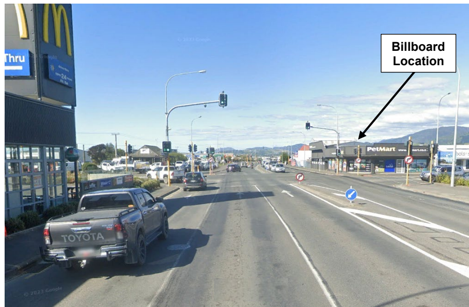
Figure 6: Gladstone Road Approach to Intersection with Lower Queen Street
