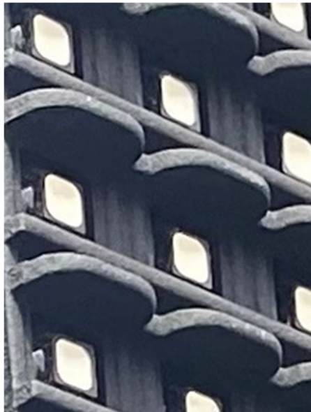
Zoomed in image of LED's and eyebrows Example LED's are at 10mm centres
