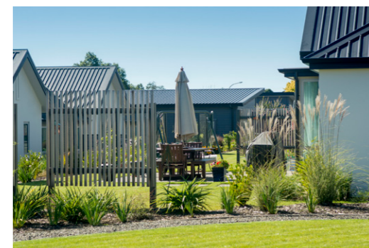
Private yard - To comply with 'TRMP' standards, allowing for 6m open spaces per lot.
