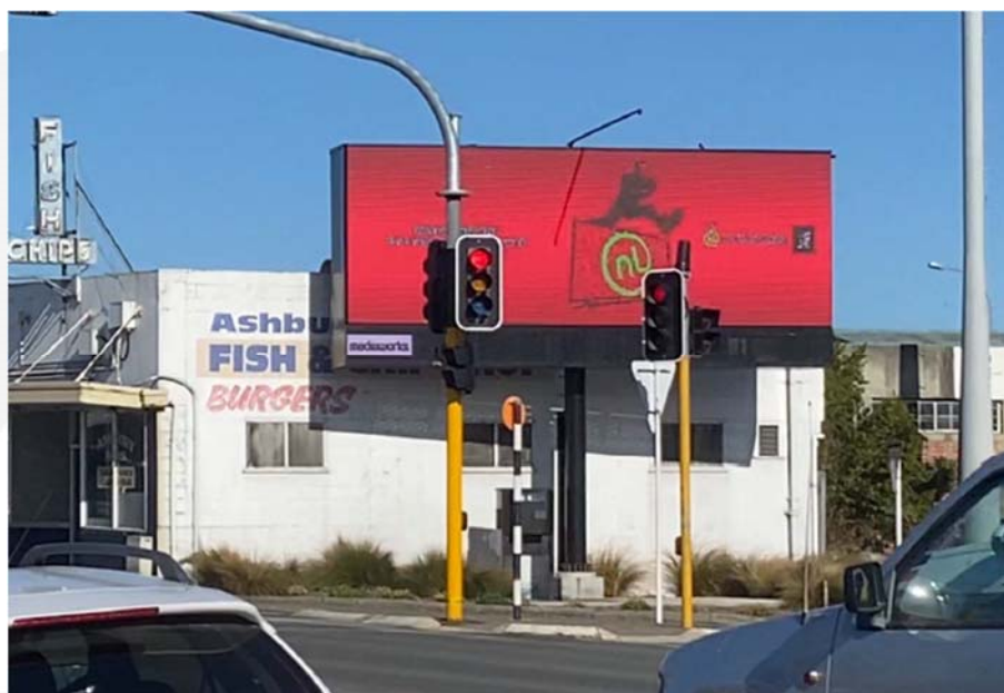
Photograph 7: Traffic Signal Overlap, State Highway 1, Timaru, Showing Visual Separation Created by Target Board
